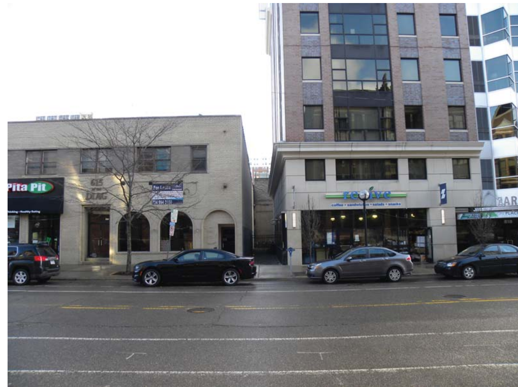
LEFT & TOP RIGHT: E. University Avenue looking southeast towards the site.
