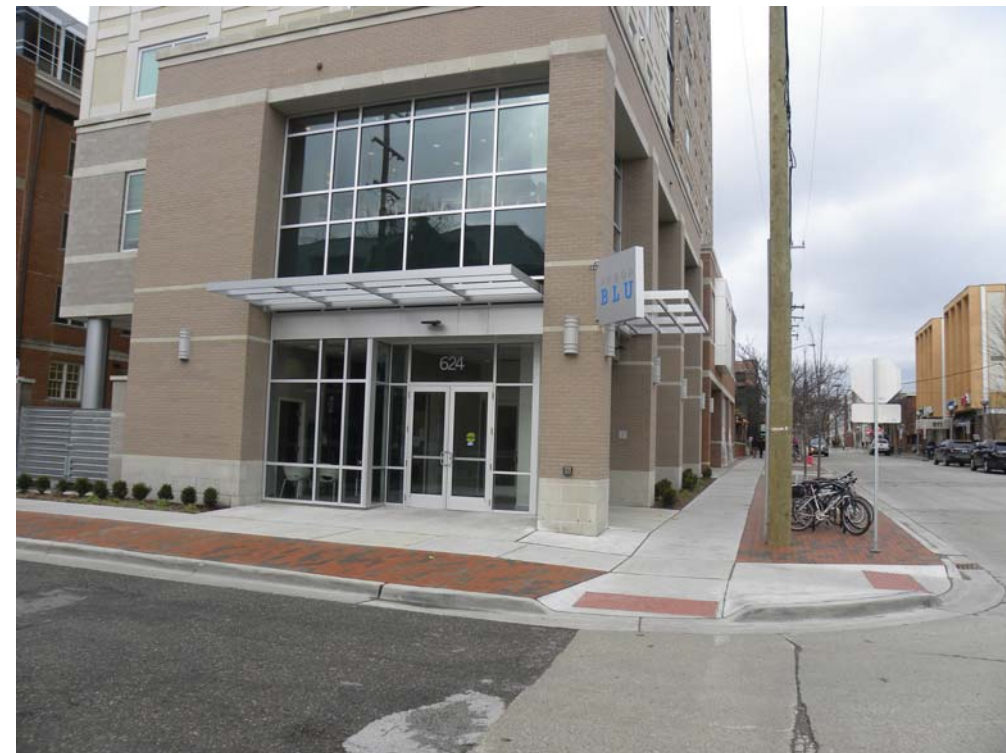
Arbor Blu located on the northwest corner of Church St. and Willard St.
