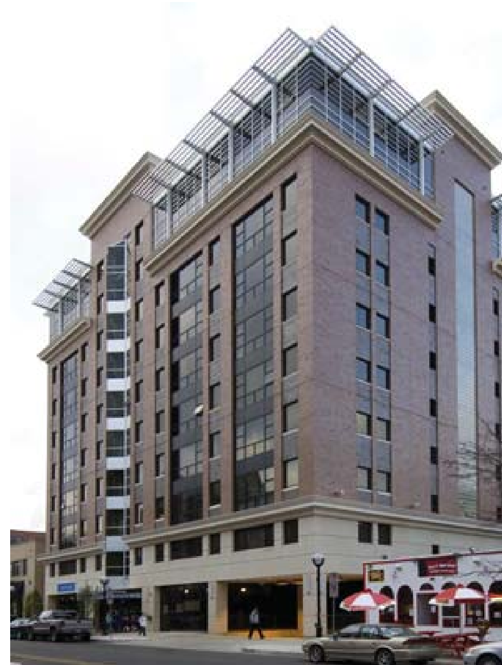
Zaragon Place located off of E. University Avenue.
