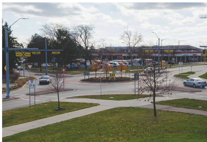
While the entire corridor will be modeled in VISSIM, RODEL will be used for detailed analysis and design of roundabouts.
