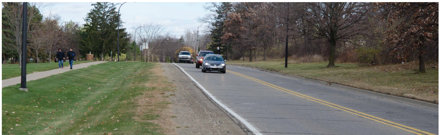
Narrow pavement lanes and lack of paved shoulders inhibit on-street travel by bicyclists. Also, the vertical terrain poses sight distance concerns when exiting some subdivisions.
