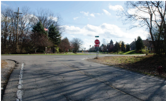
Dhu Varren Rd and Green Rd are offset, creating two T-intersections.
