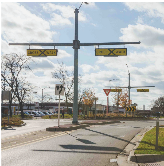
Enhanced signs, lighting and pavement markings can improve pedestrian safety at key crossing locations.
