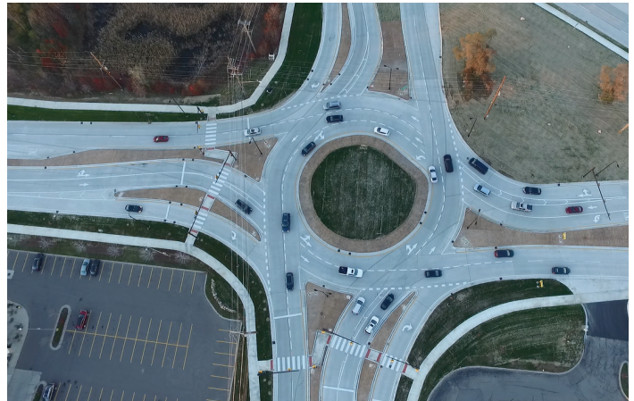
Example of snagged right-turn bypass lanes.
