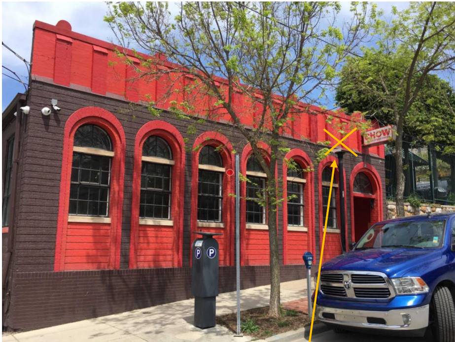
Photo of Existing Condition (one awning over each of 6 windows)
