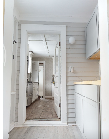
VIEW OF INTERIOR OF BREEZEWAY. ORIGINAL CLAPBOARD SIDING CAN BE SEEN AT SHARED KITCHEN WALL. SOUTH WINDOWS ARE DRYWALLED OVER AND CABINETS BLOCK WINDOWS.
