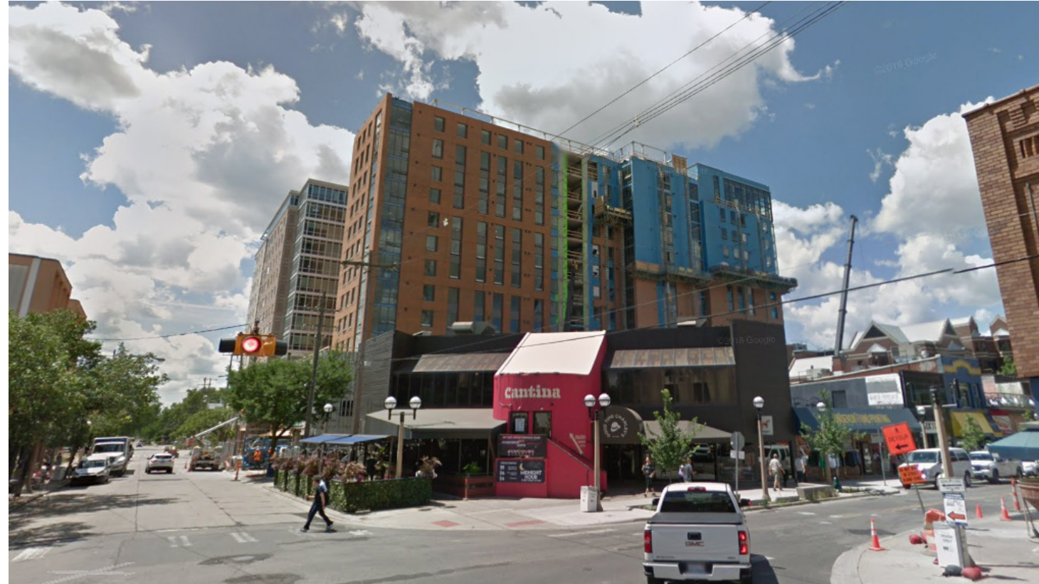
STREETVIEW OF SITE - LOOKING SOUTHWEST
