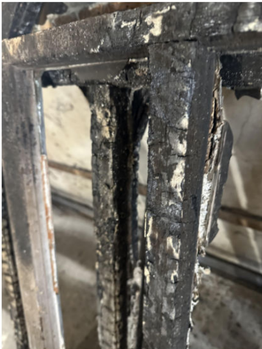
(E) WINDOW SASHES (FIRE DAMAGED)
