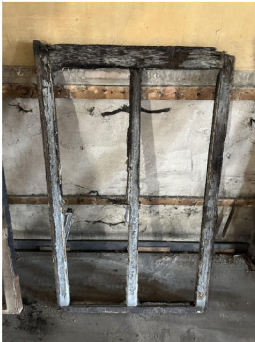
(E) WINDOW SASHES (FIRE DAMAGED)
