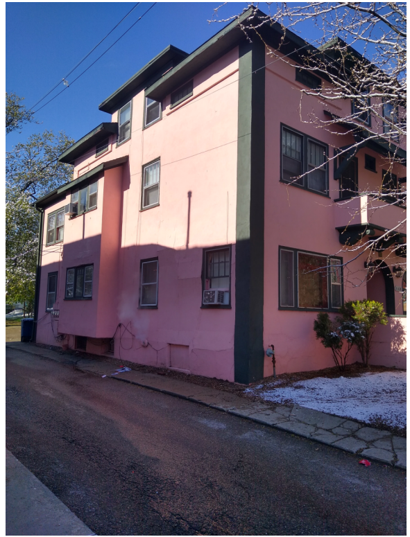
Existing NorthEast facade
