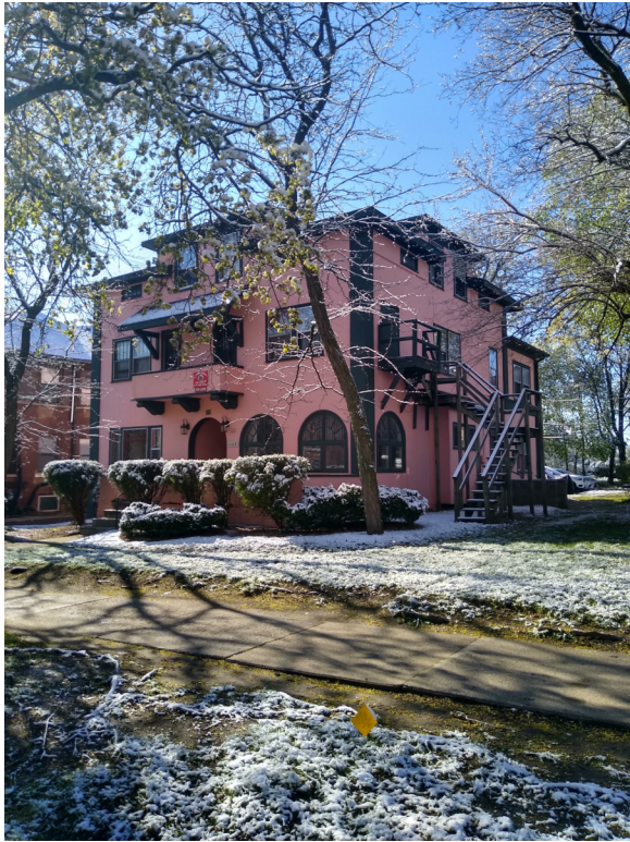
Existing North facade - facing Hill Street
