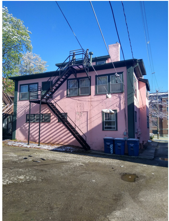
Existing South facade - facing parking
