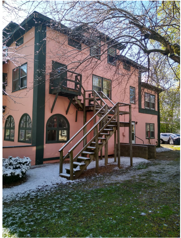
Existing NorthWest facade
