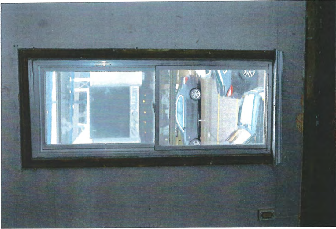
INTERIOR OF SECOND FLOOR EAST WINDOWS
