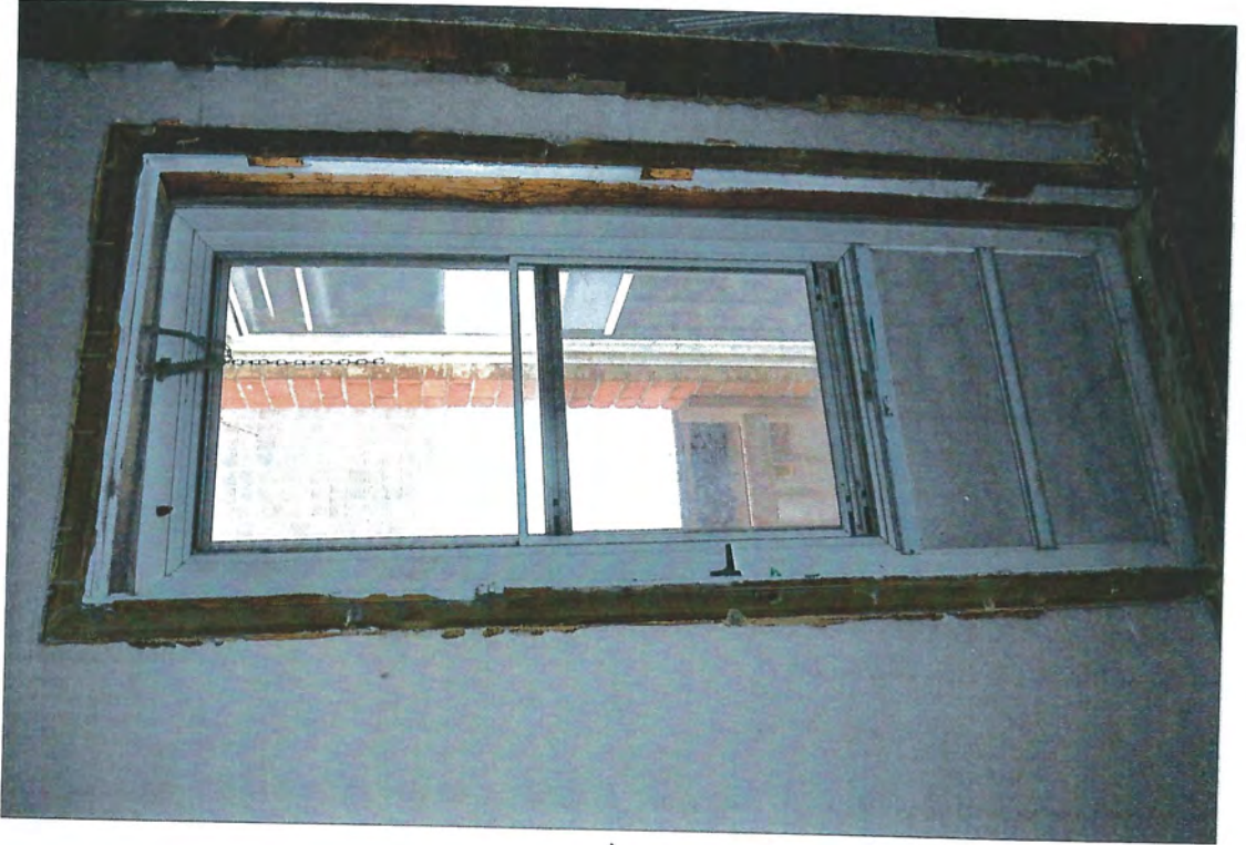
SOUTH-EAST BALCONY DOORWAY
