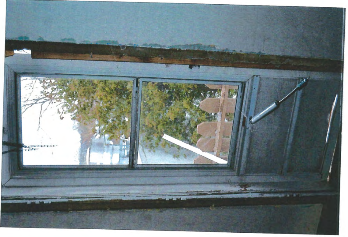
WEST BALCONY DOORWAY
