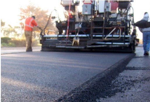
Pavement Resurfacing
