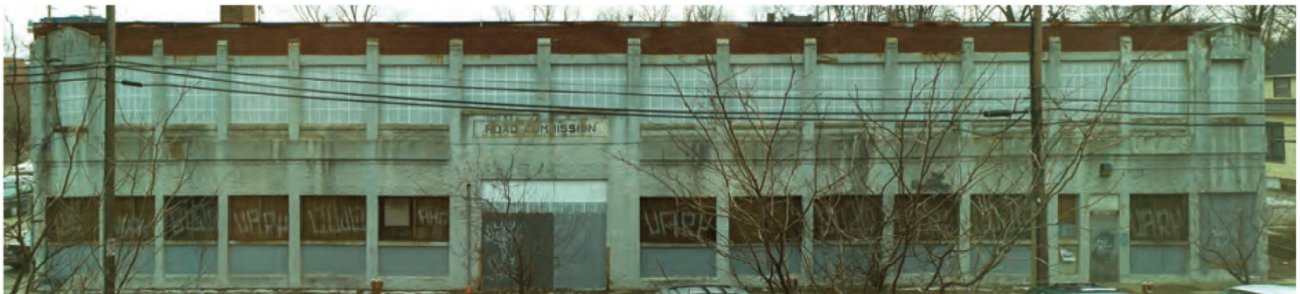
P10. North Façade, 2013 Assessment Photo
