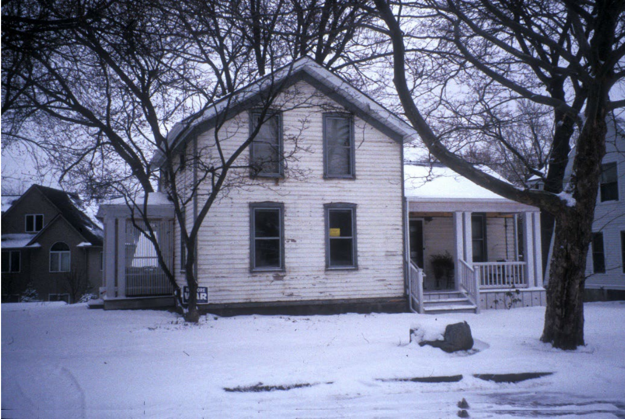
543 Detroit Street (2004 File Photo, taken shortly after aluminum siding was removed)
