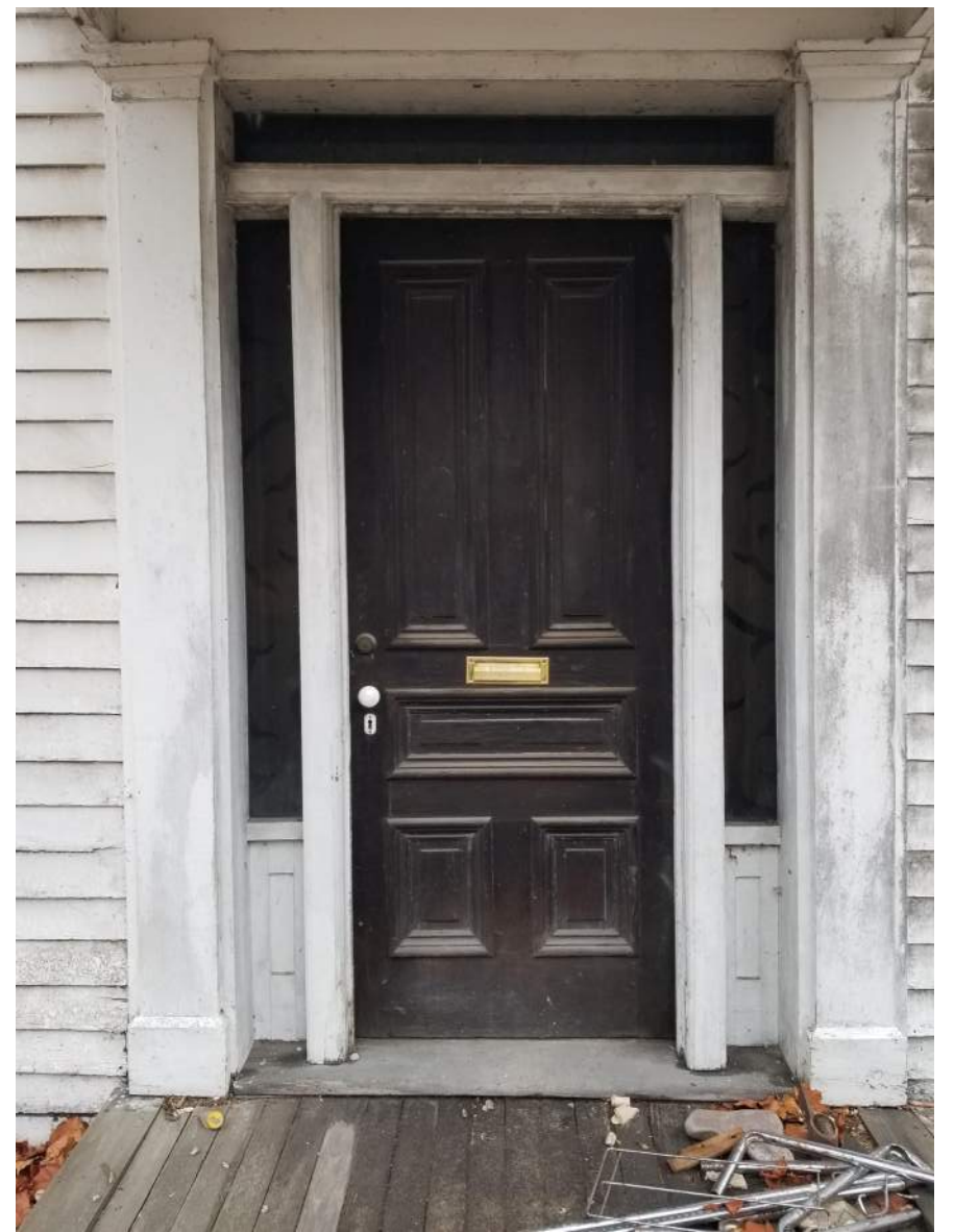
Existing front door
