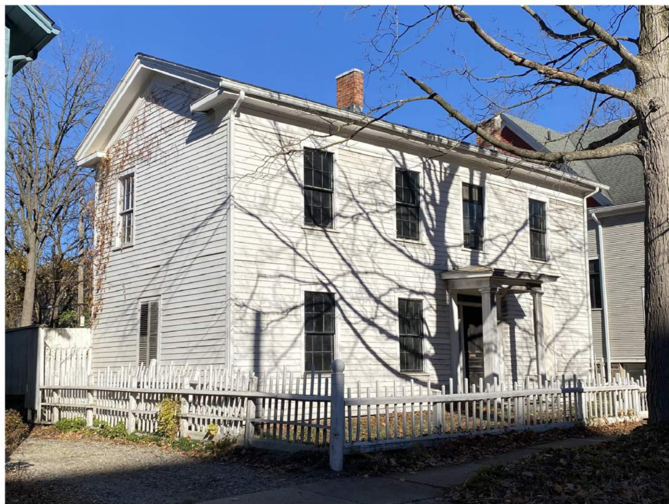
View of Existing South Elevation
