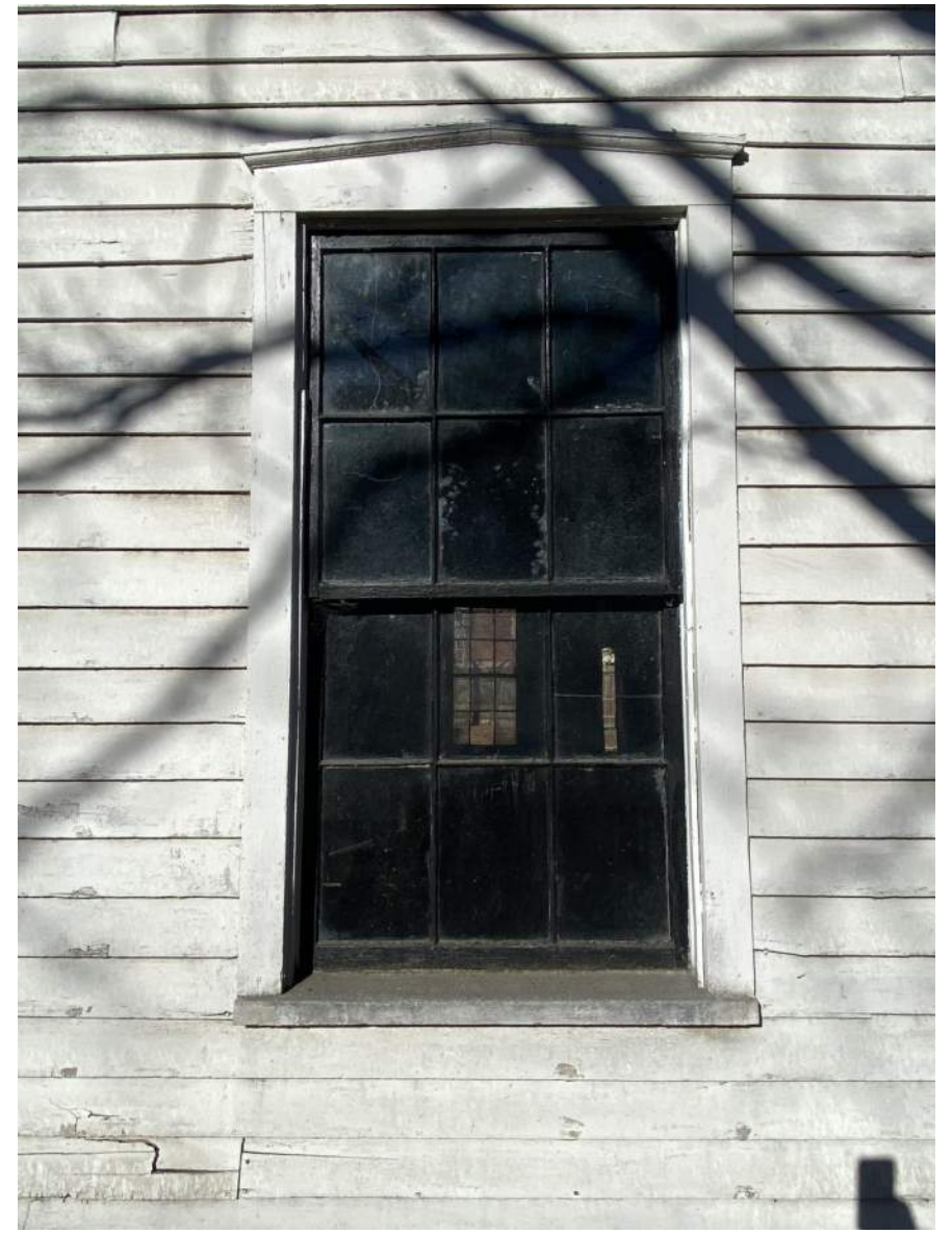
Existing window - DH-A
