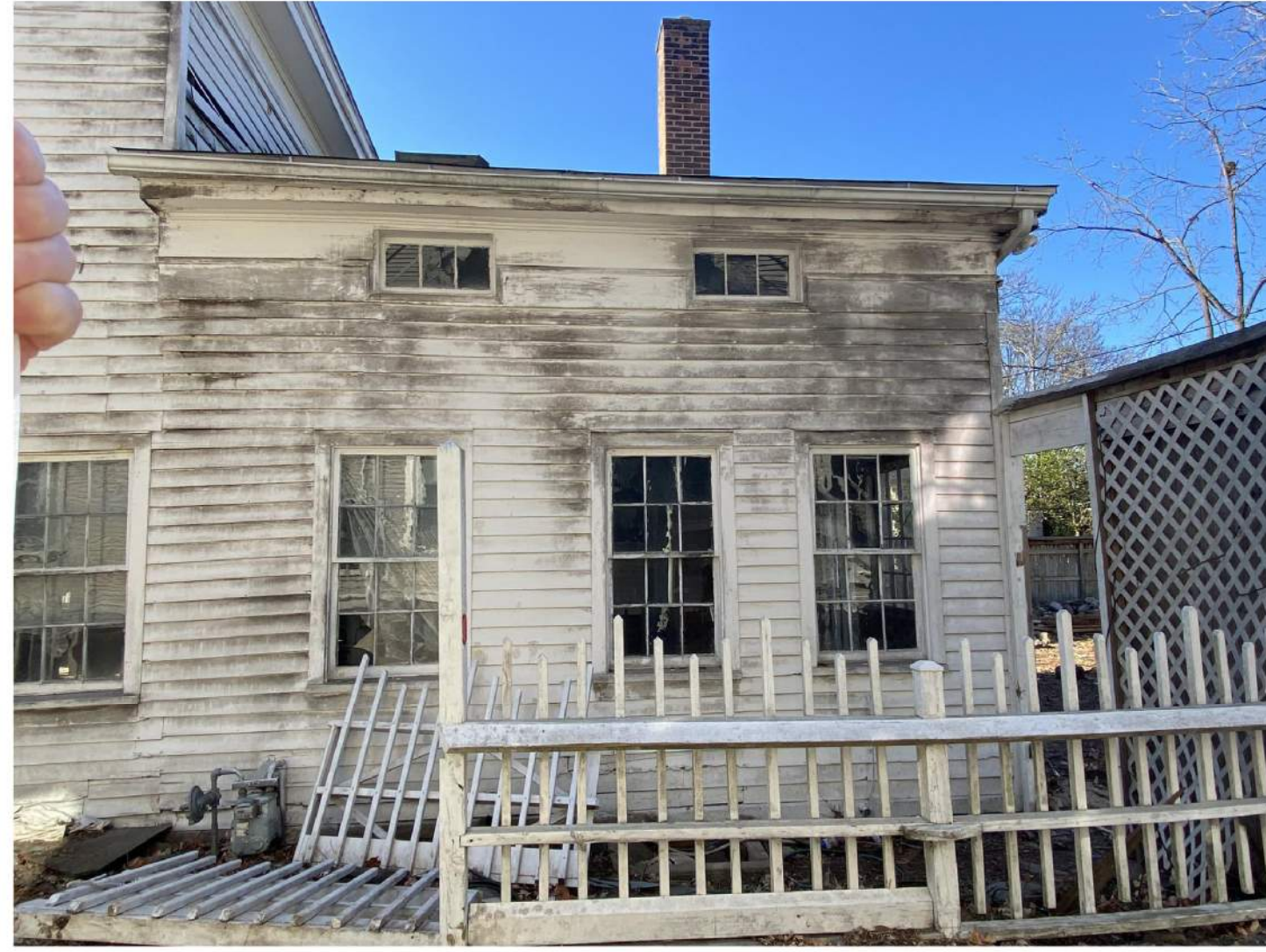
View of Existing East Elevation
