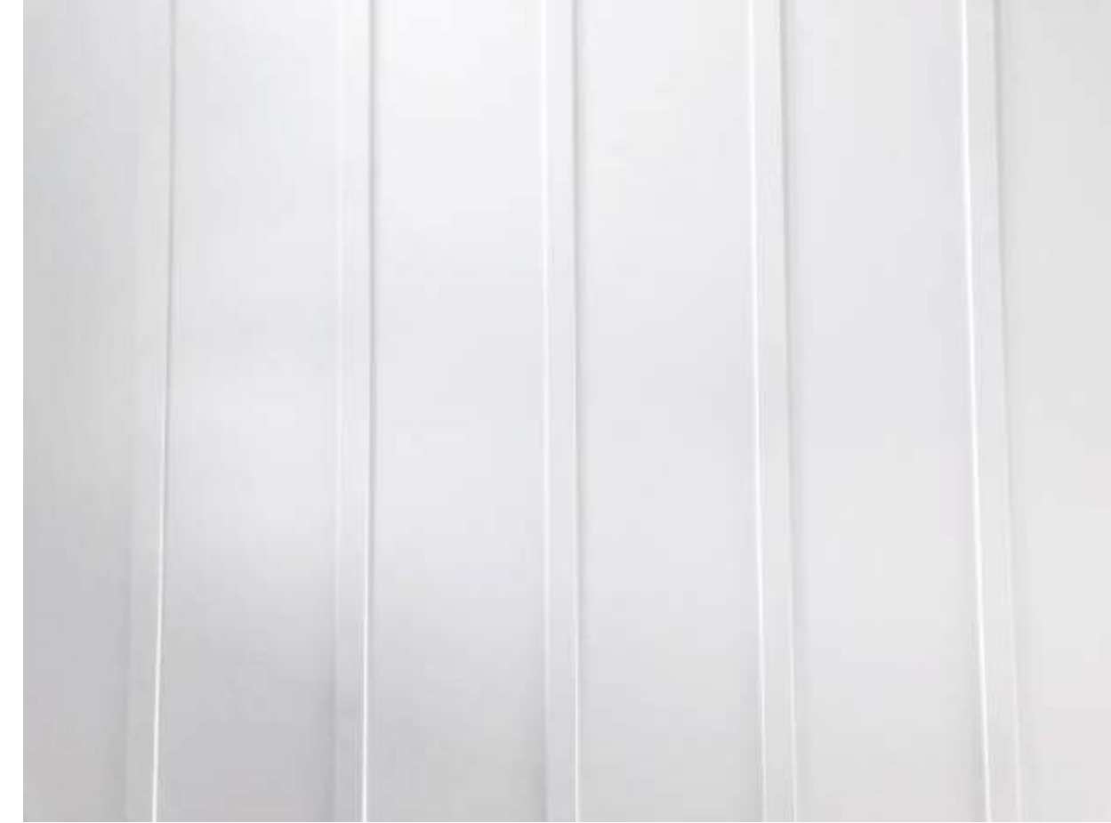
White board-and-batten vertical siding
