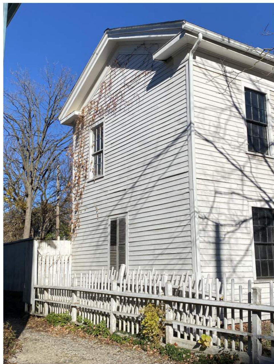
View of West elevation
