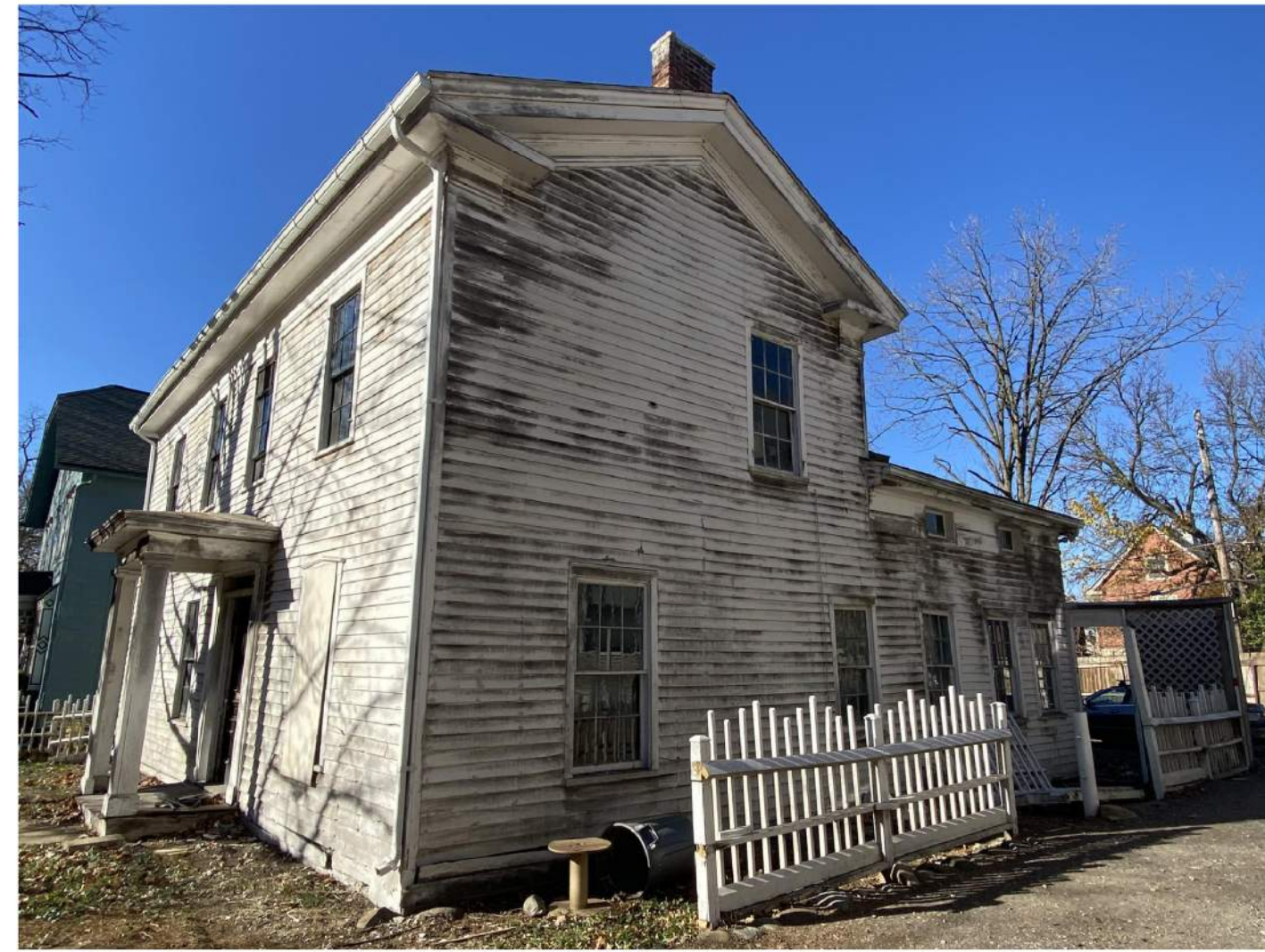
View of Existing East Elevation
