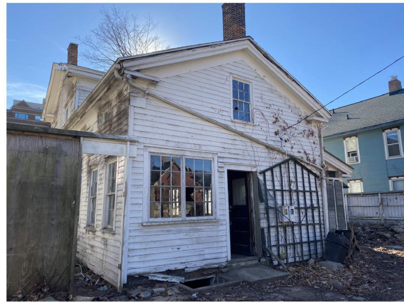
View of Existing North Elevation
