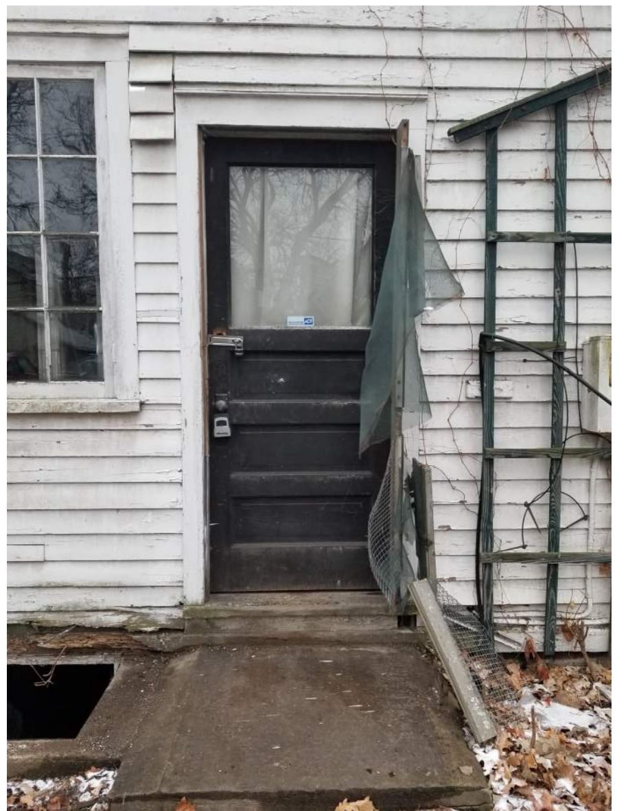
Existing back door - suspected not to be of historic significance
