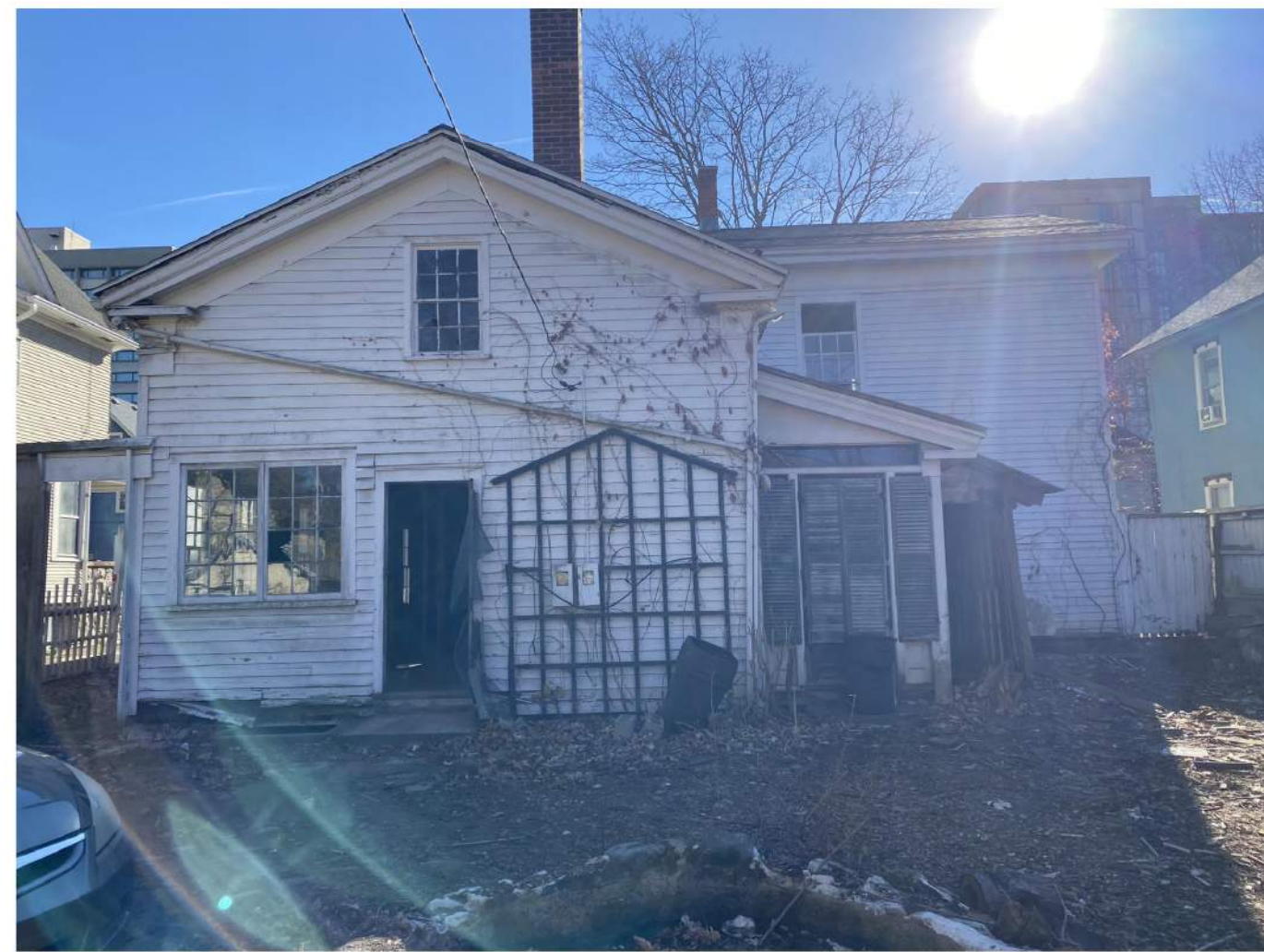
View of Existing North Elevation
