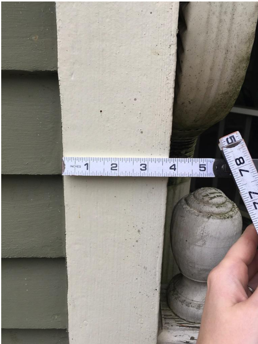
PHOTO OF EXISTING WOOD CORNER BOARD PROPOSED FIBER CEMENT CORNER BOARDS TO BE 3 1/2" W/ SMOOTH FINISH
