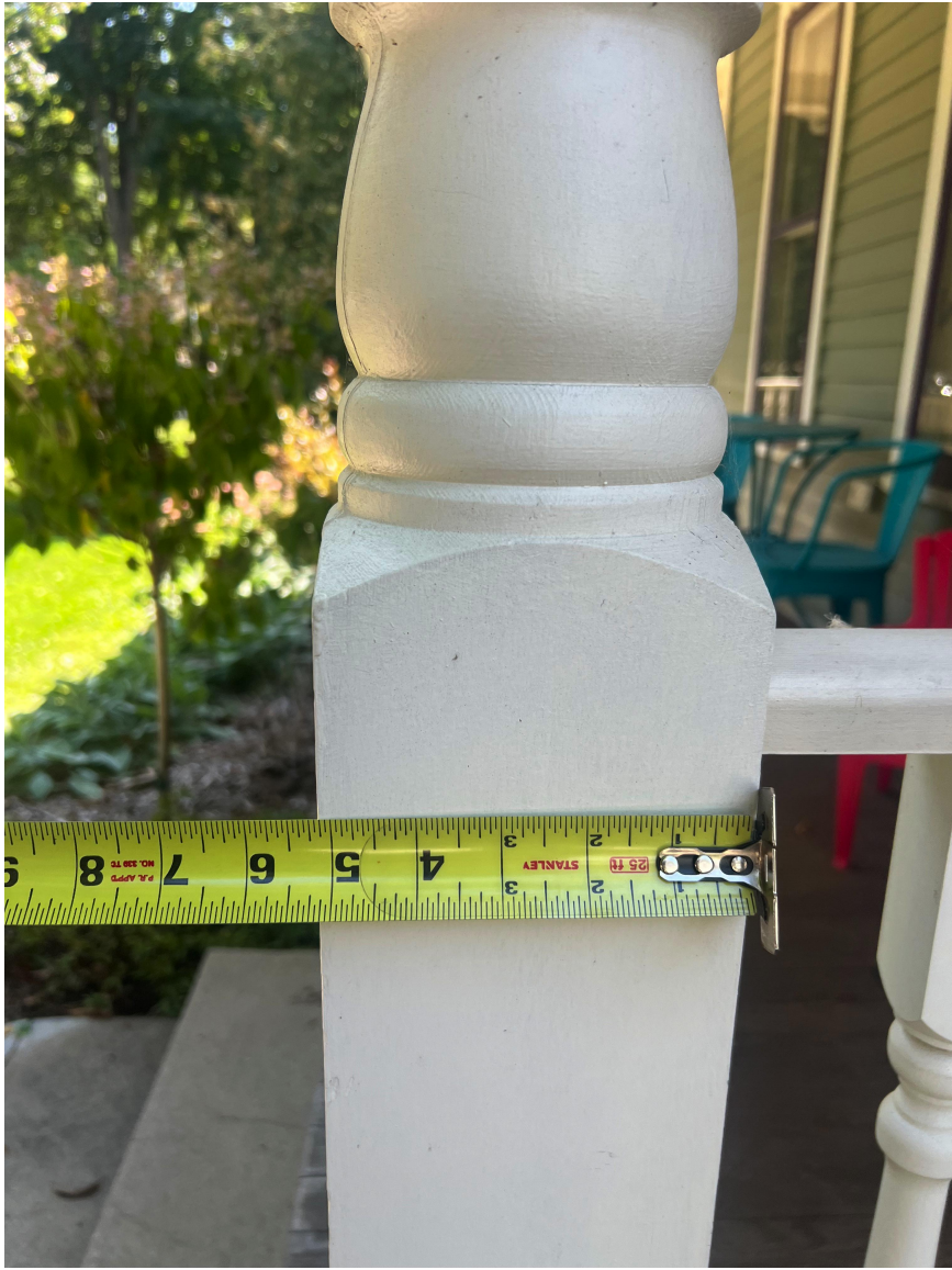
PHOTO OF EXISTING FRONT POCH COLUMN. NEW COLUMNS TO BE 6"
