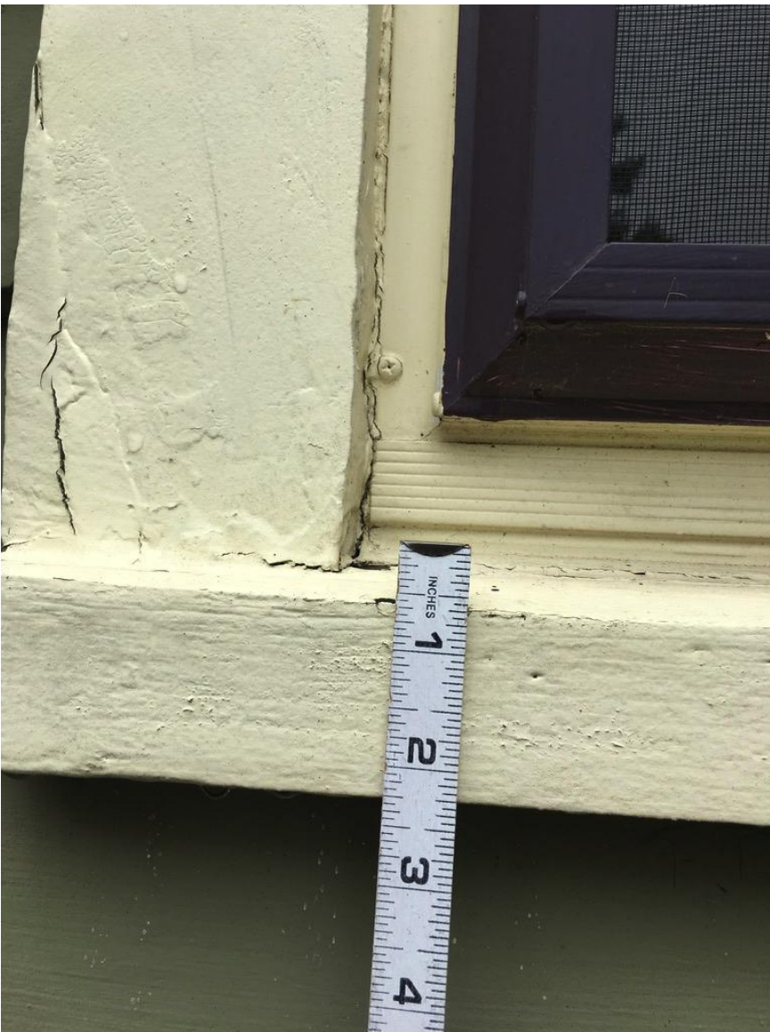
PHOTO OF EXISTING WOOD WINDOW SILL PROPOSED SMOOTH CEDAR SILL TO BE MAX. 2"
