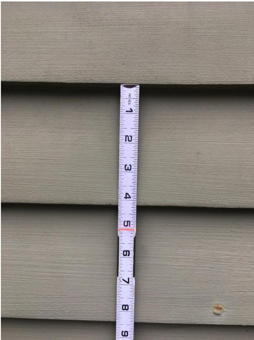
PHOTO OF EXISTING WOOD LAP SIDING PROPOSED FIBER CEMENT LAP SIDING TO HAVE 4" MAX. EXPOSURE & WOOD GRAIN FINISH
