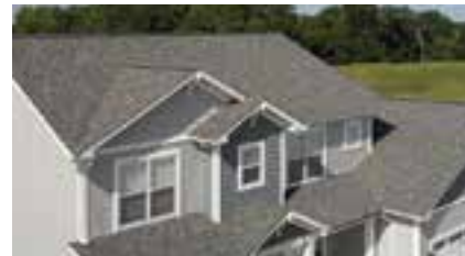
ROOFING AND VENTILATION
