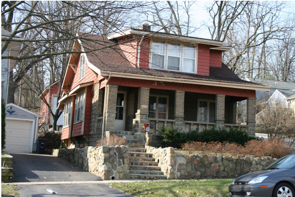
Image 1: 415 West Mosley Street (2008 staff photo)
