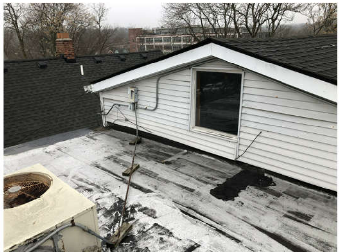
(E) EAST VIEW OF ROOF
