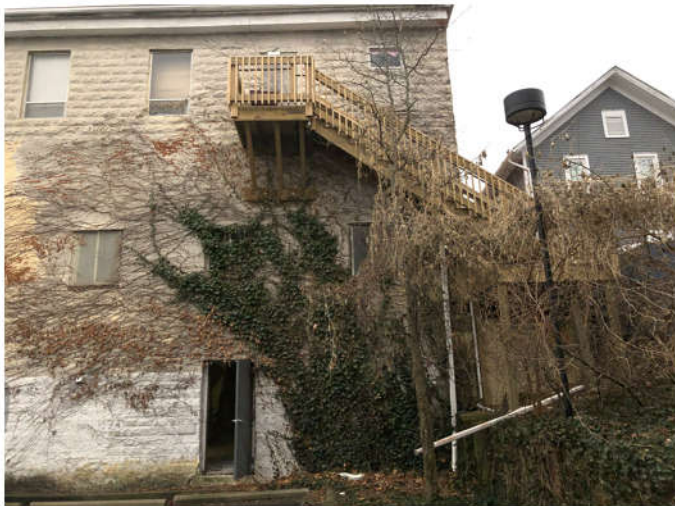
(E) WEST REAR VIEW
