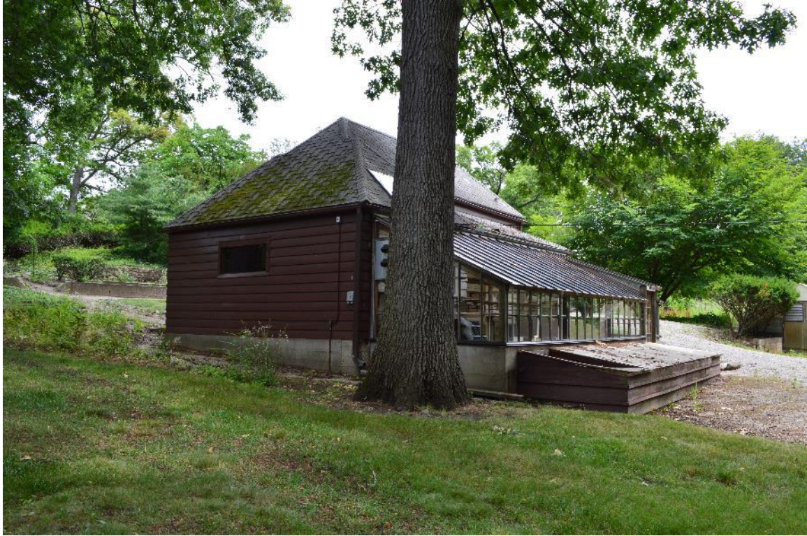
Looking northeast at shop and greenhouse, July 2017
