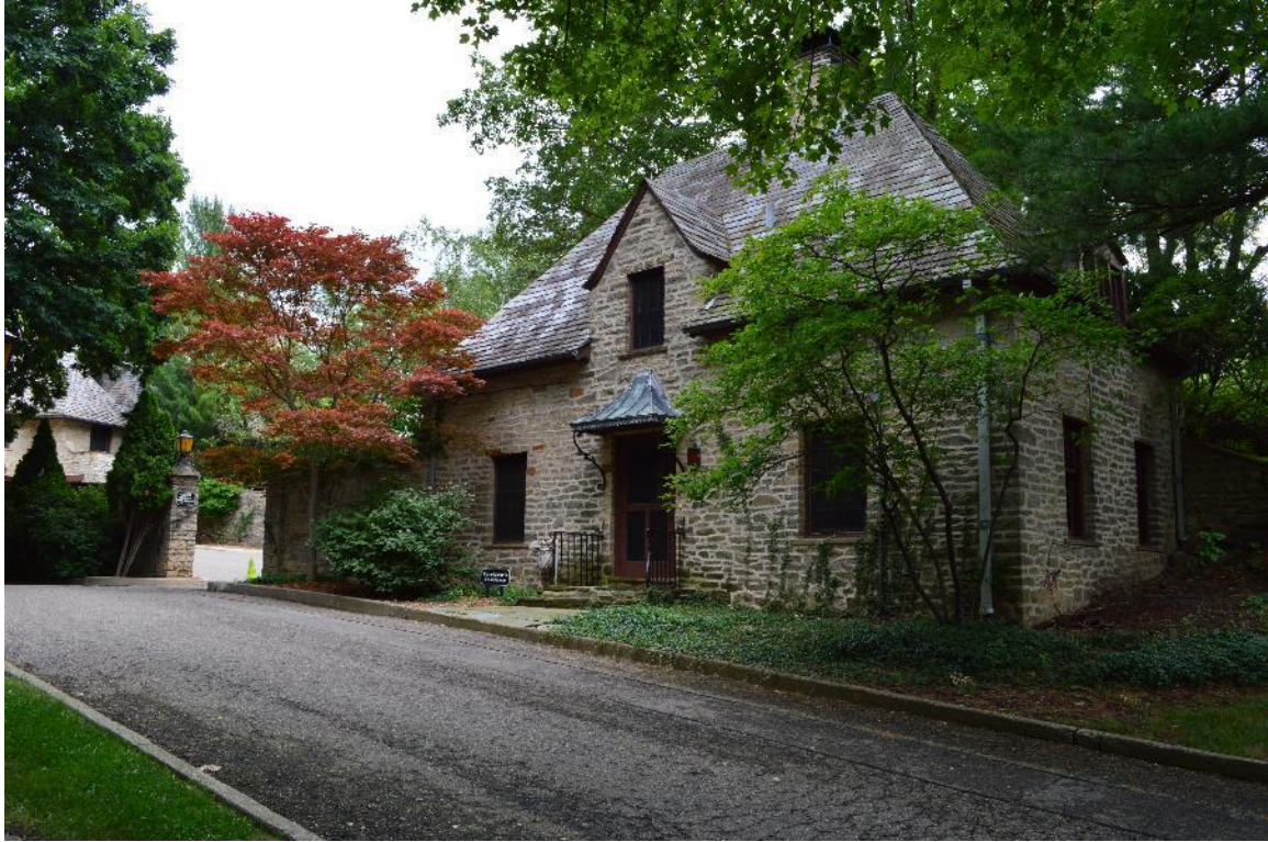
Looking northeast at caretaker's cottage with house to left, July 2017
