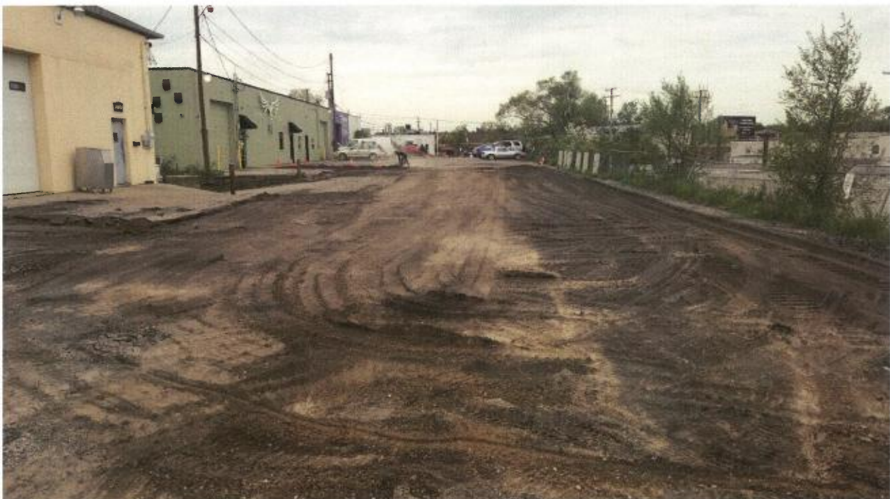
Tear out of existing degraded asphalt.
