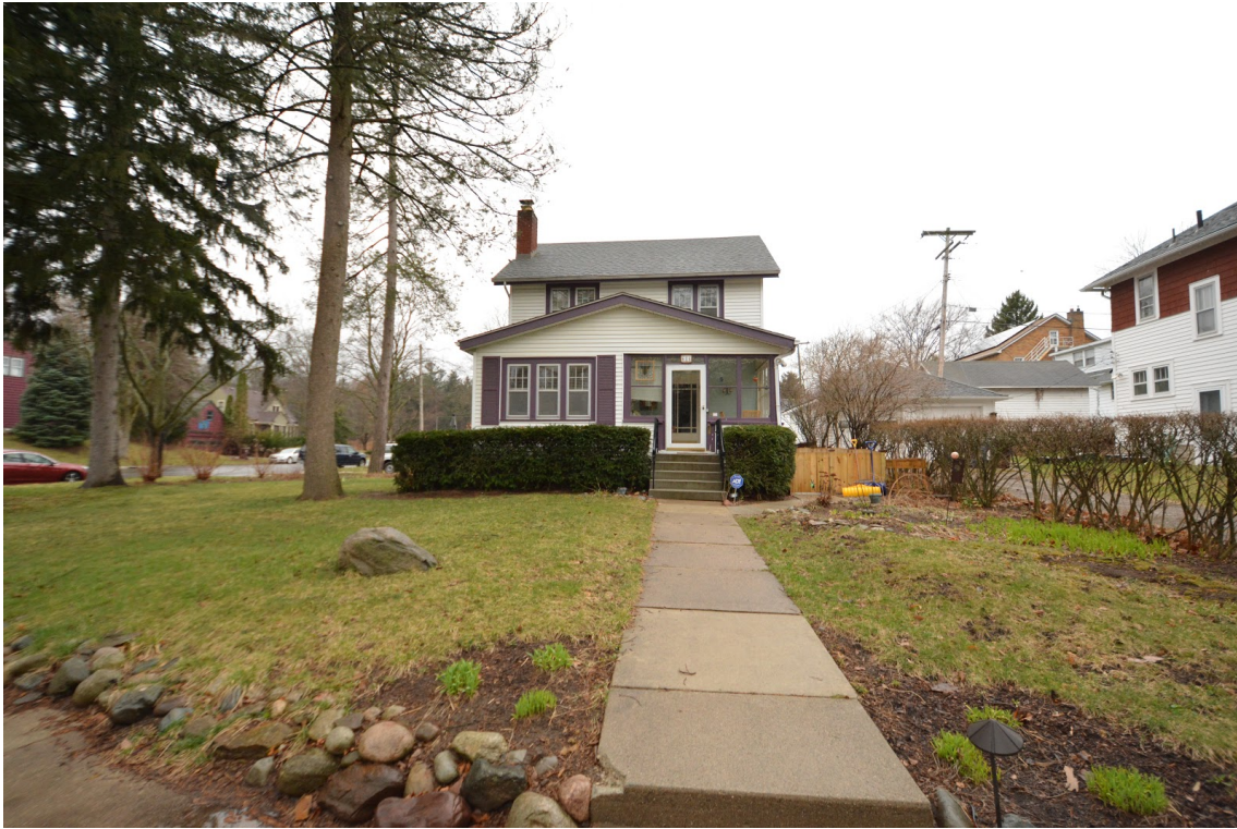
Front entry on Soule Blvd.
