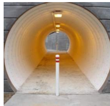
Completed tunnel example
