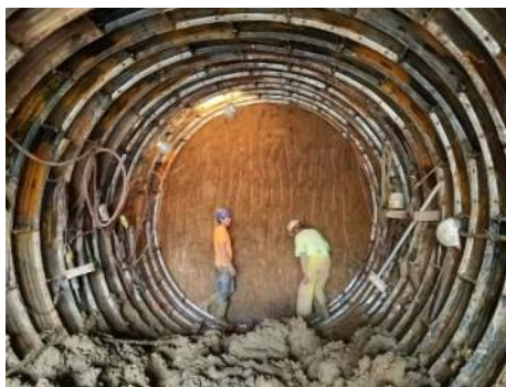
Hand digging to install tunnel
