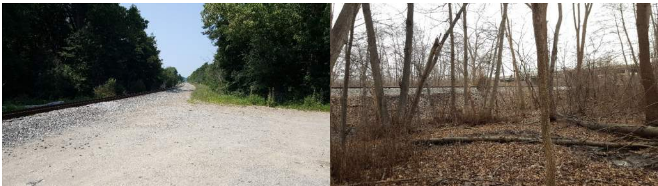
Exhibit 1-3: Existing site looking west at north side of tracks (left) and looking north from south of tracks (right)
