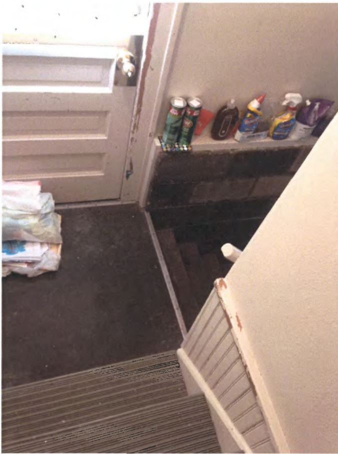
EXISTING STAIR LANDING & EXTERIOR DOOR @ BASEMENT STAIR
