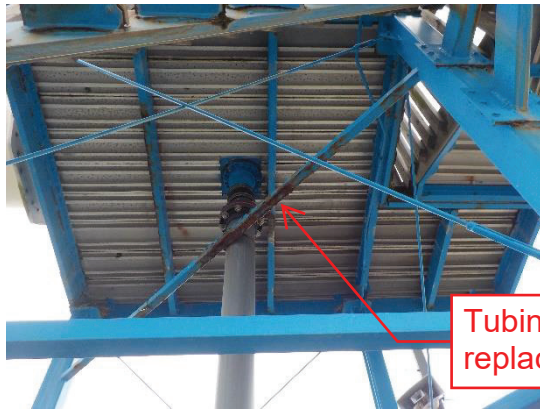
2" X 2" STEEL TUBE AT WATER STACK (TO BE REPLACED)
