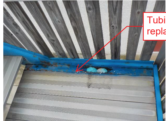
3" X 1½" STEEL TUBE AT LANDING (TO BE REPLACED)
