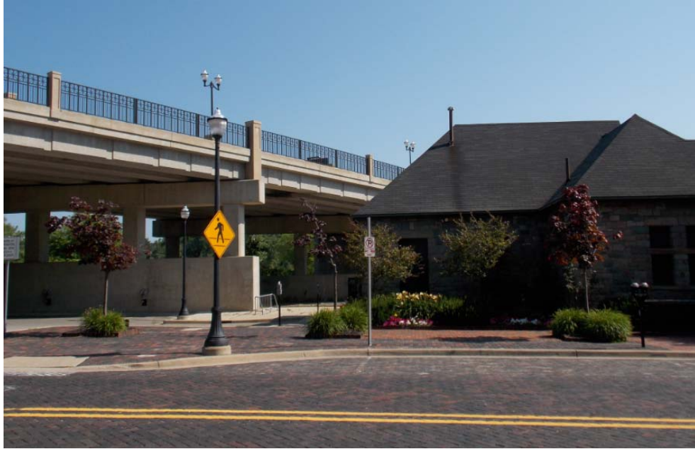
Plate 2: Looking northwest toward the MCRR westernmost ancillary building and the Broadway Street Bridge from Depot Street parking area
