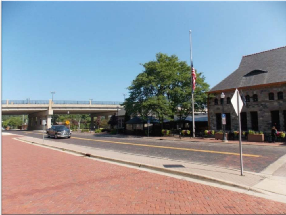
Plate 1: Looking northwest toward Depot Street; MCRR to the right with the Broadway Street Bridge in the background
