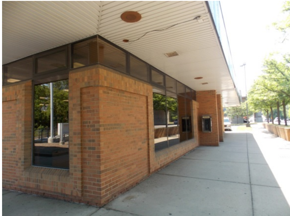
Plate 3: Looking east toward the south elevation of the Amtrak Station along Depot Street; Broadway Street Bridge in the background
