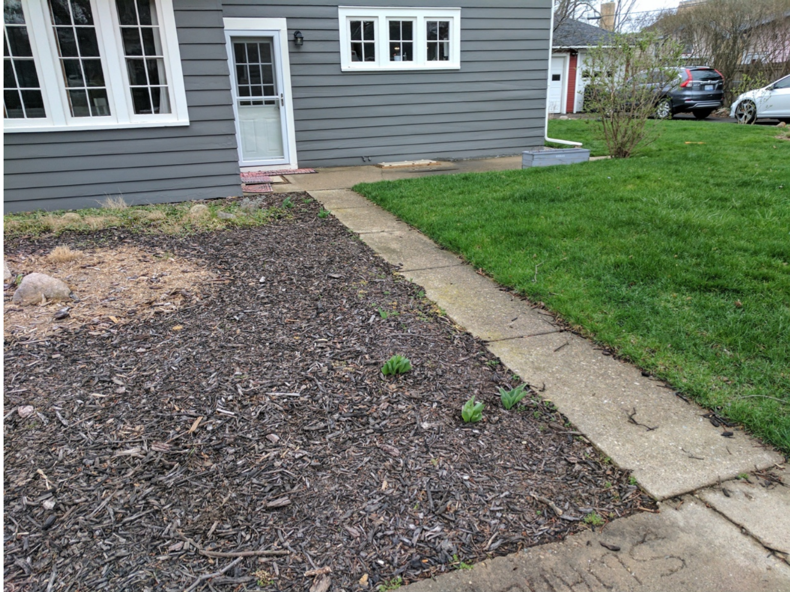
West (Cement Walkways & Pad)
