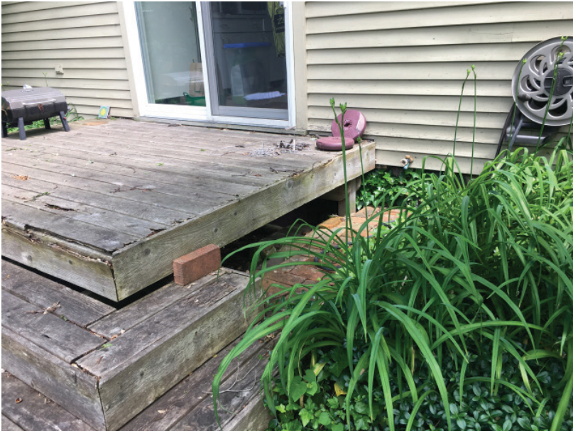
Closeup of Existing Deck
