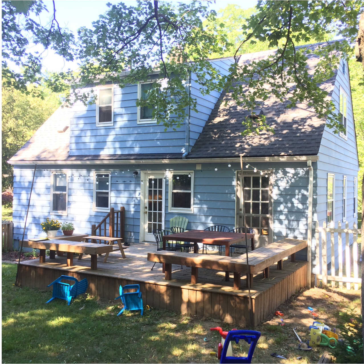
EXISTING HOUSE - SIDE OF PROPOSED REAR YARD ADDITION NOT FOR CONSTRUCTION
