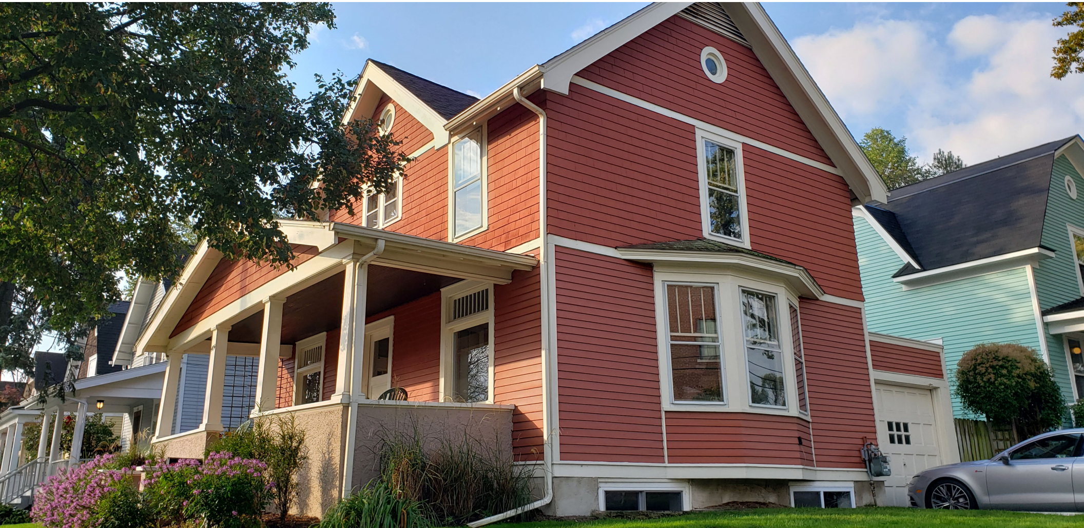
Northeast corner of house looking south Note: recently installed handrails not pictured
