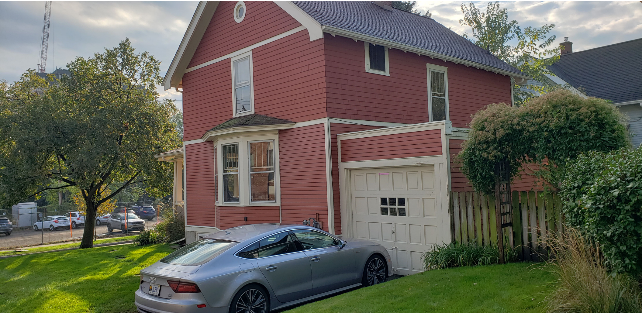
Northwest corner of house looking southeast: Proposed location of new Upper Addition
