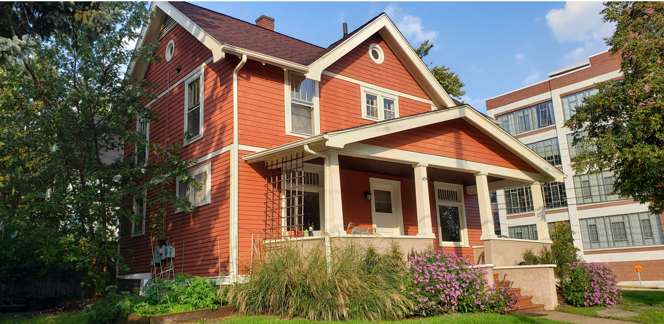
Southeast corner of house looking northwest Note: Recently installed handrails not pictured
