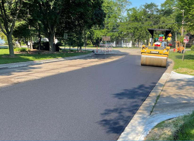
Local Street Paving on Crestland Drive
