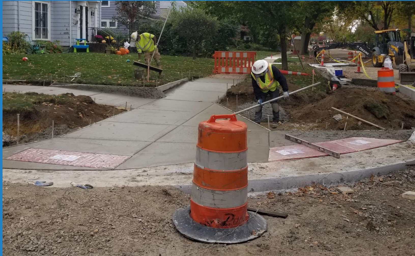
ADA Sidewalk Installation on Granger Ave.
