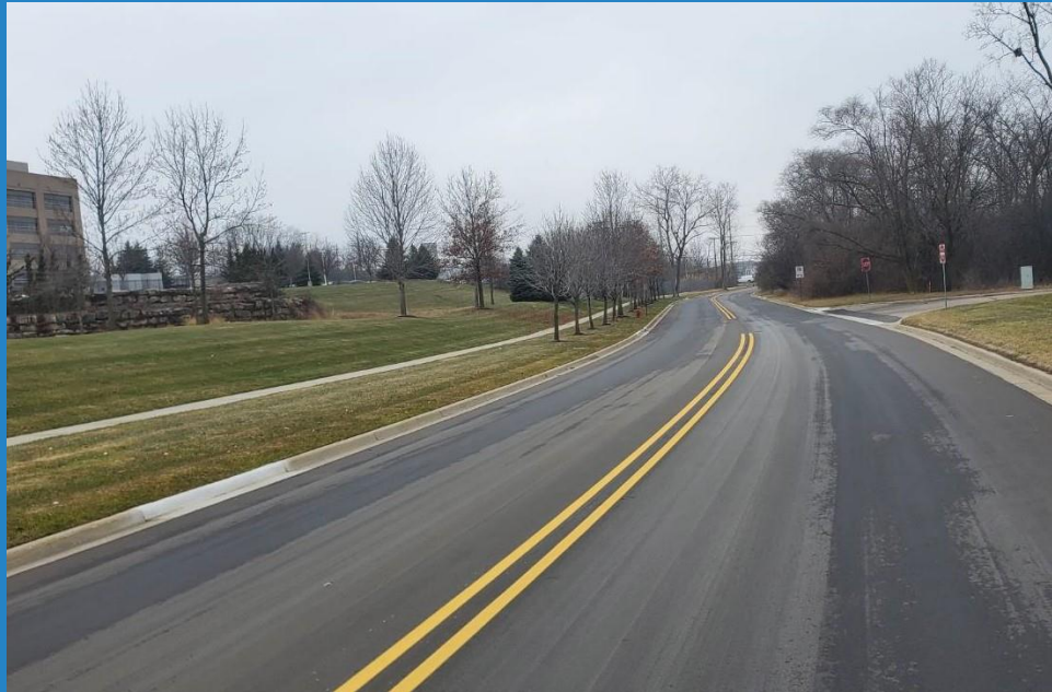
Street Resurfacing on Boardwalk Drive
