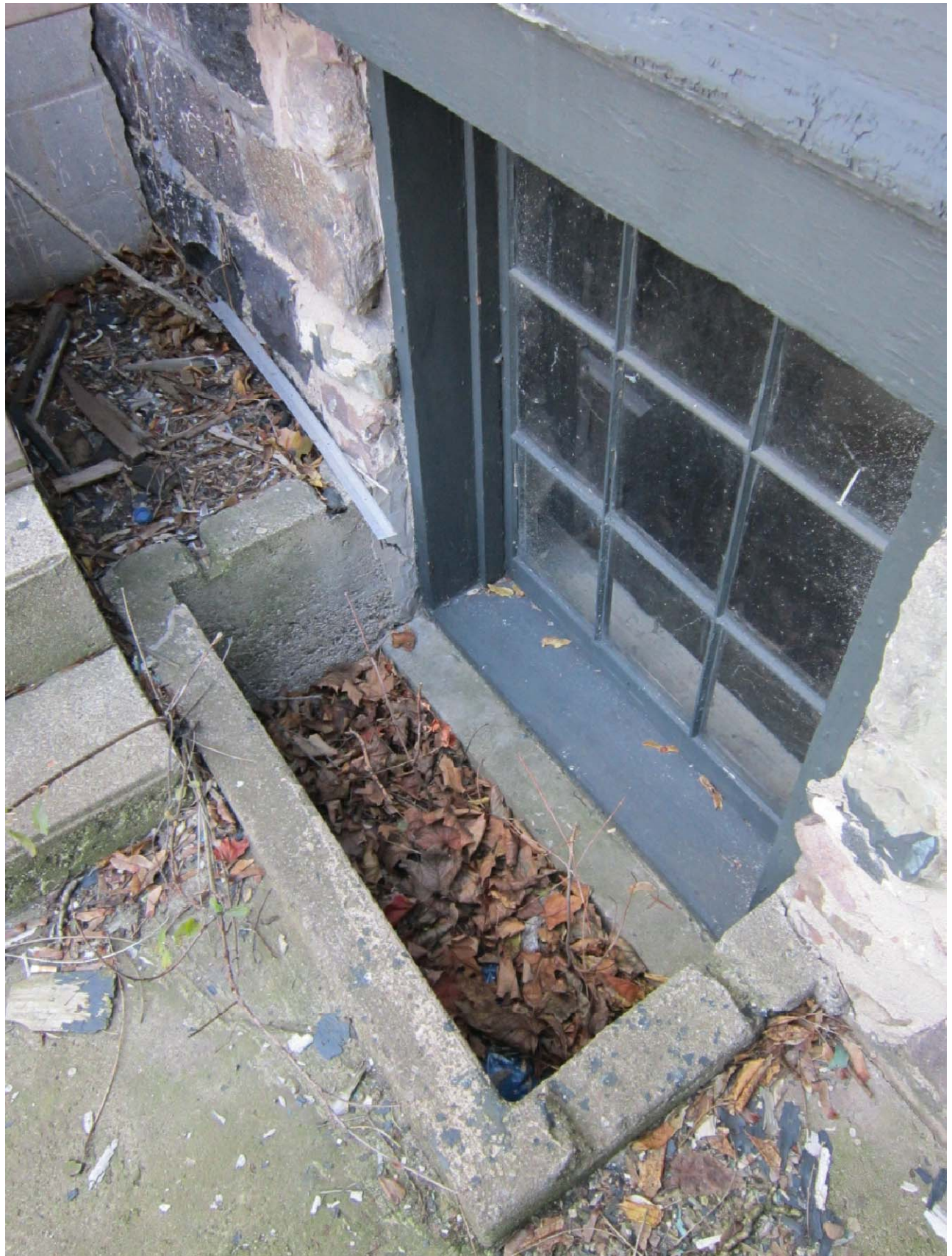
DETAIL OF BASEMENT WINDOW
