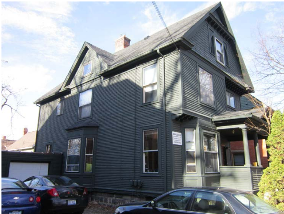
SOUTH AND EAST
