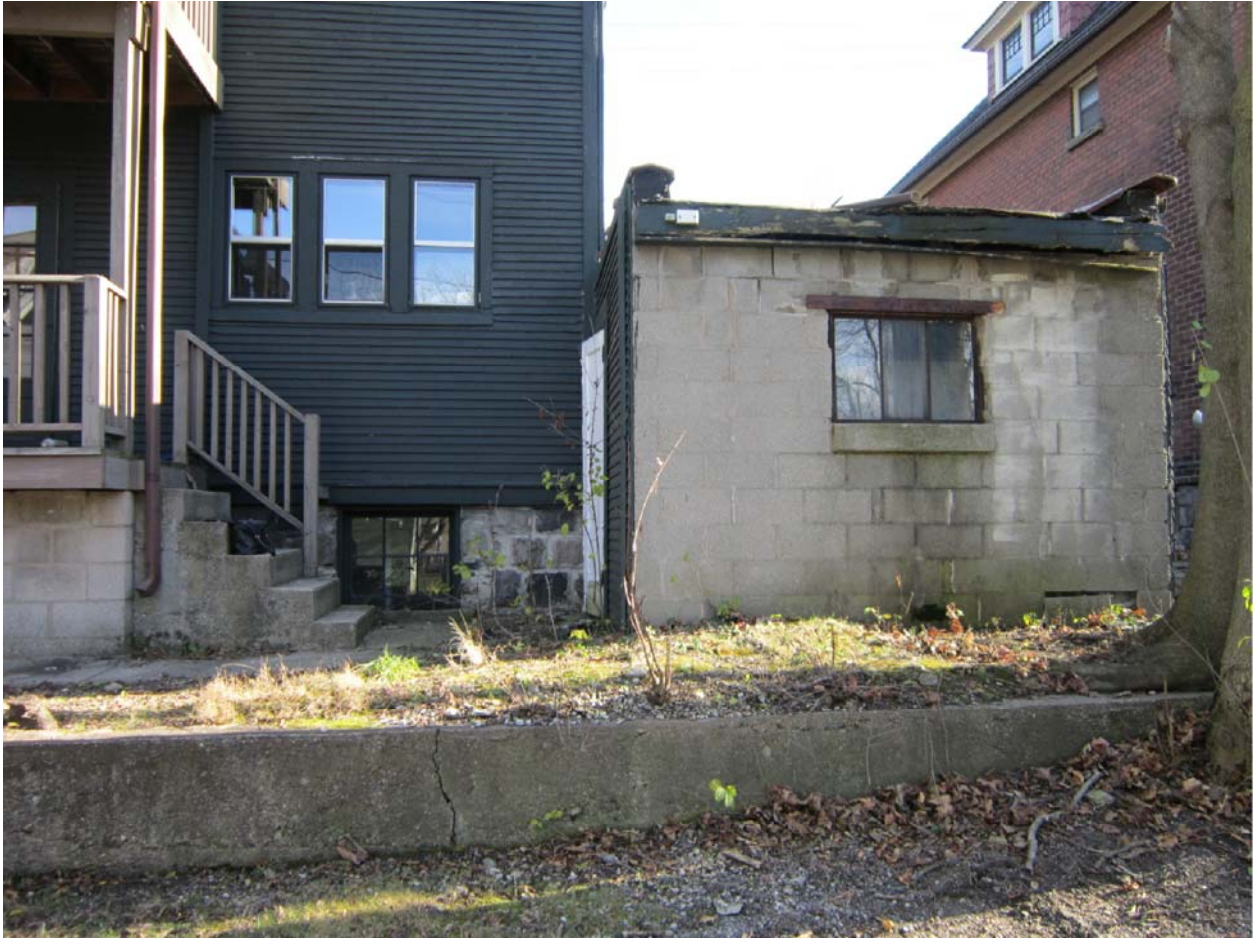
REAR FACADE (partial)
