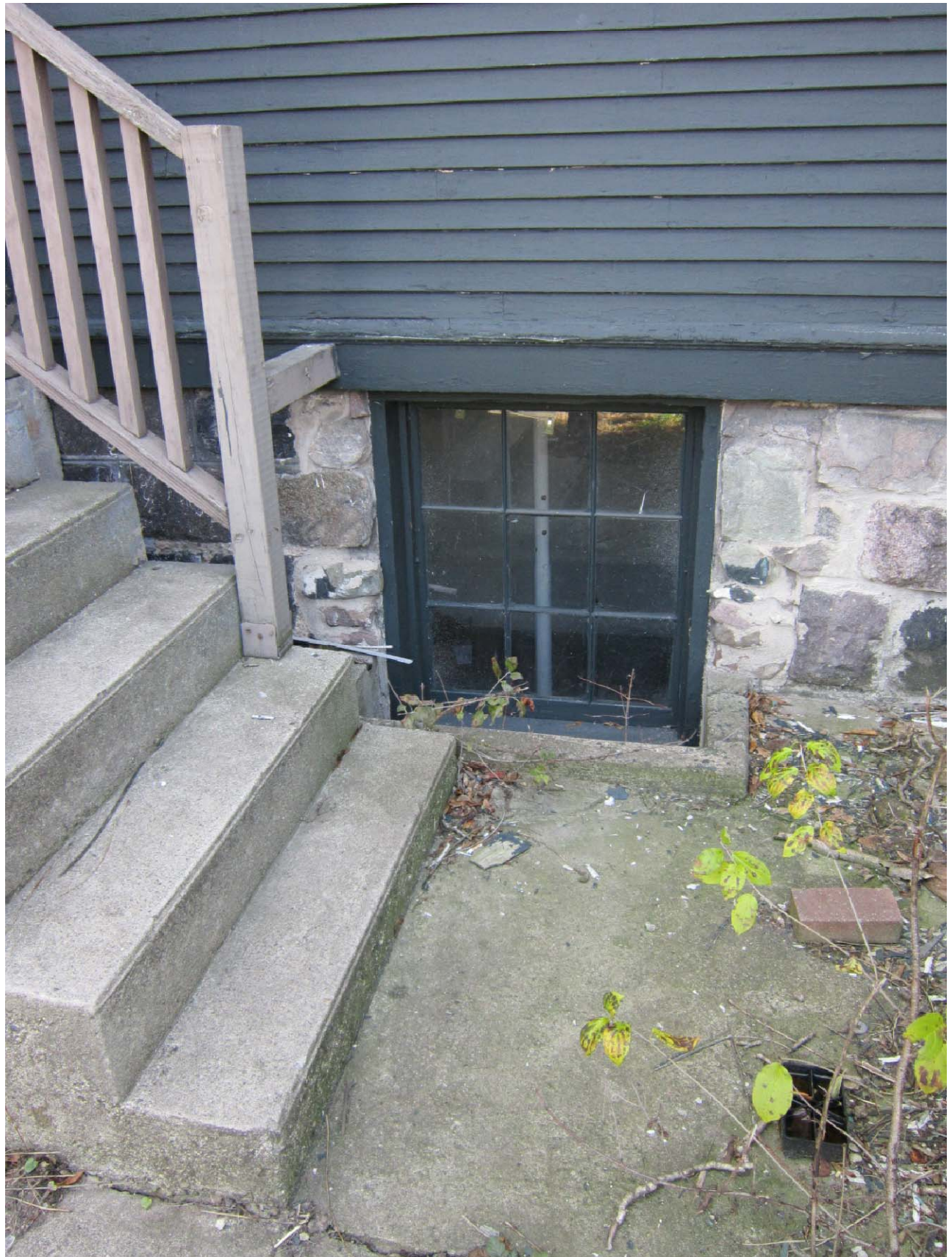
DETAIL OF BASEMENT WINDOW
