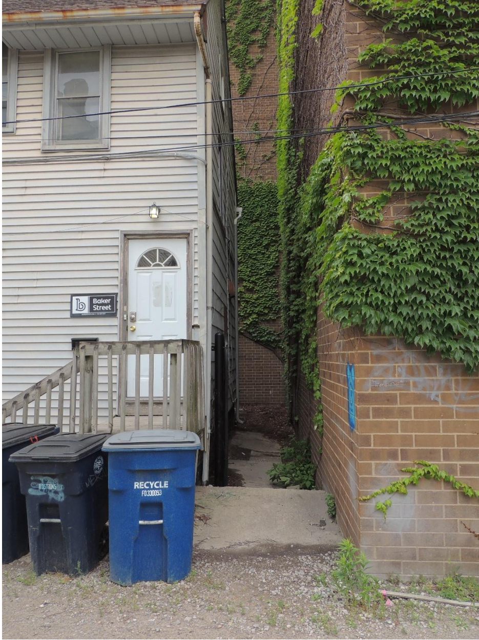
VIEW OF BARRIER FREE RAMP ENTRY POINT ON THE EAST SIDE OF 311 EAST LIBERTY. THIS ALLEY IS 4'10" WIDE AND FORMS THE REAR YARD OF 311. THE BUILDING TO THE RIGHT IS THE 7 STORY SOLID UNFENESTRATED BRICK FASCIADE OF 301 EAST LIBERTY. 301 OWNS 10 INCHES OF THIS 4'10" ALLEY.
