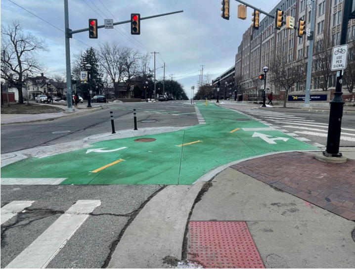
Protected biking intersection with curb and green pavement markings
