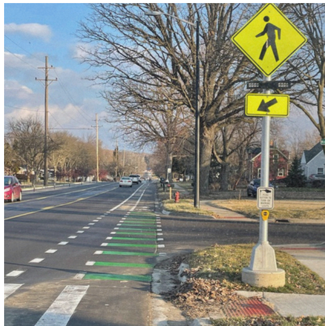
Platt Rd. - Resurfacing
