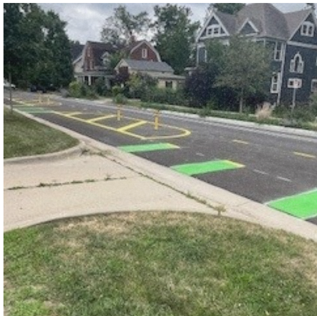
Fifth Ave. - Resurfacing
