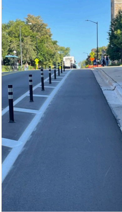
Protected Bike Lane State St.
