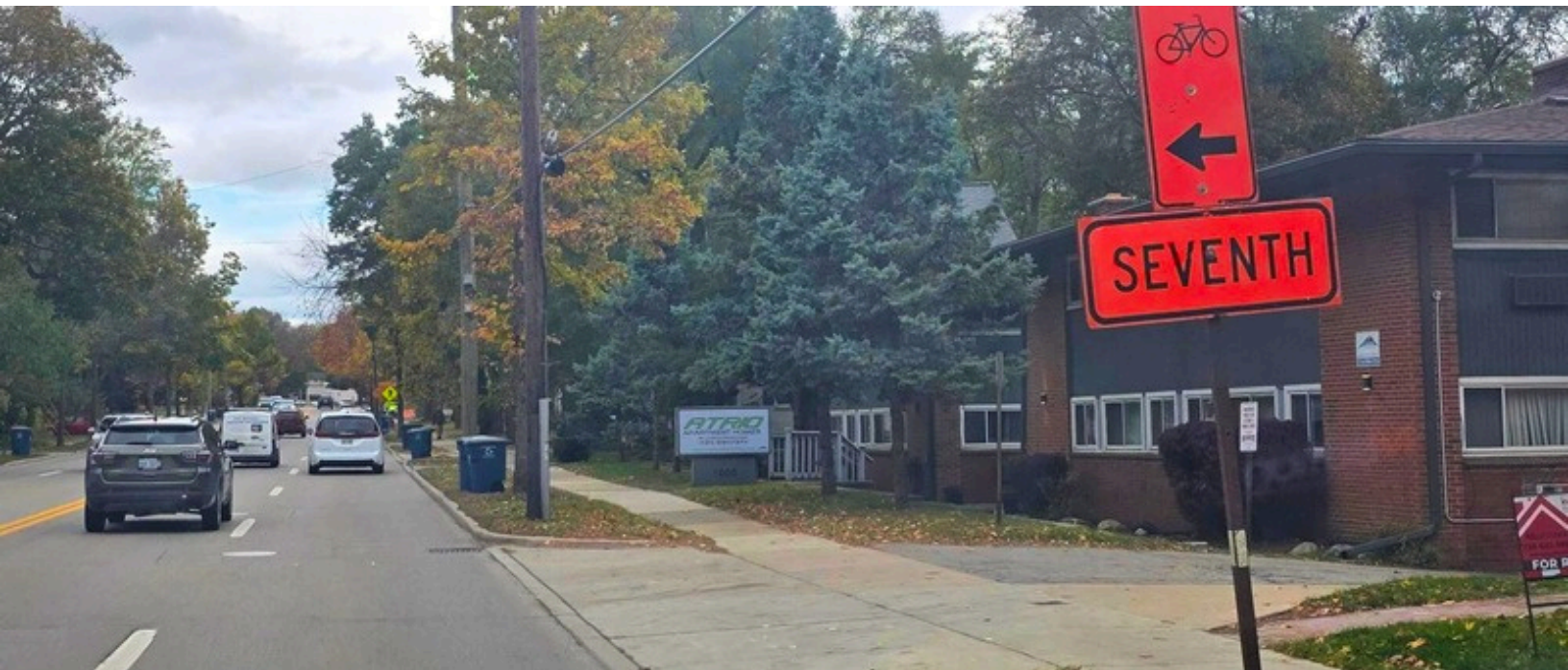
Bicycle maintenance of traffic for the Seventh St. resurfacing project.
