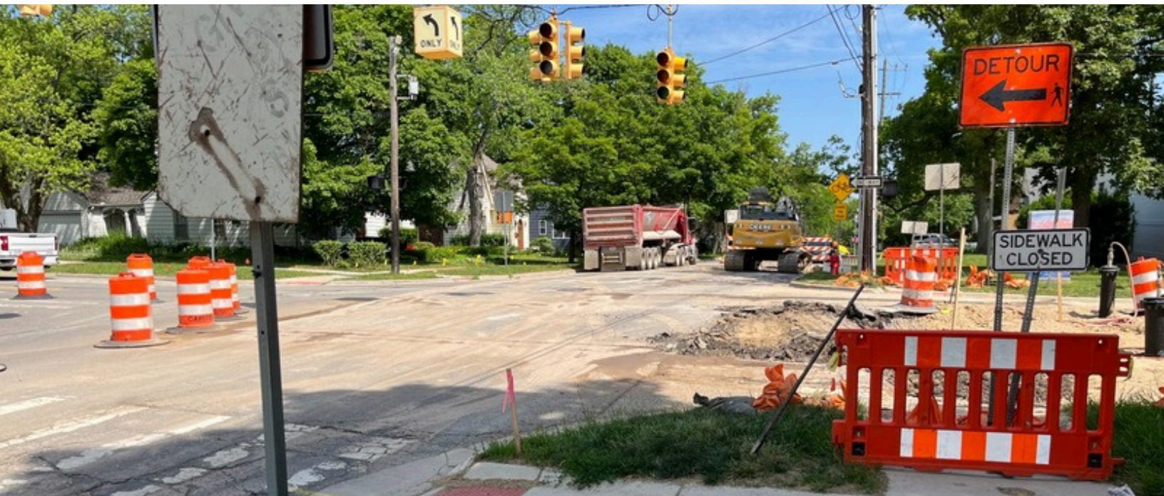
Pedestrian maintenance of traffic for the Pauline Blvd. resurfacing project.
