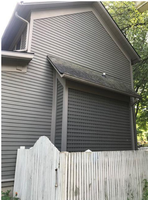
North bump out to be removed.
