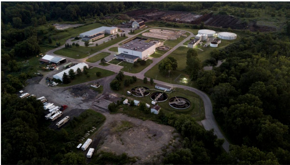
Aerial photo of the Wixom Wastewater Treatment Plant, Aug. 9, 2018.
