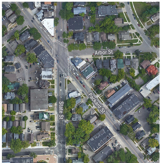
Opportunities to improve safety will be evaluated at the unique intersection of Packard and State with multiple approaches.
