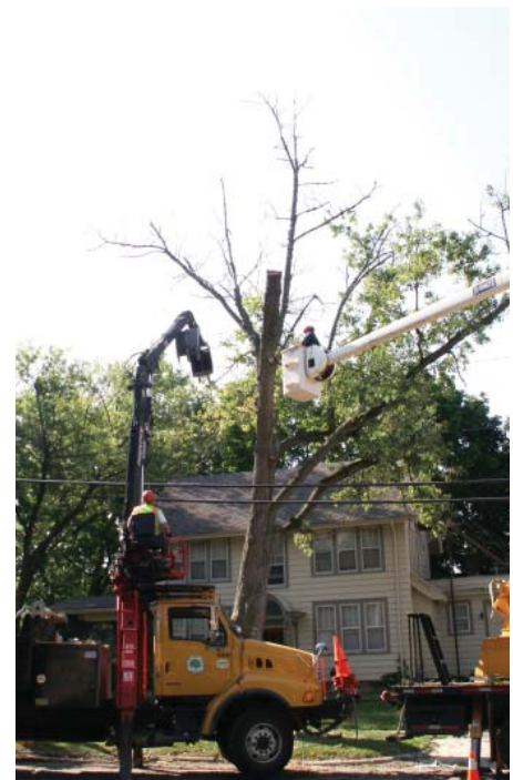
City Forestry crew removing a tree (2009)
