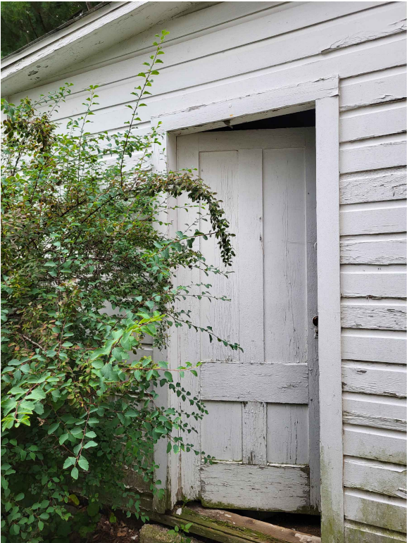
existing garage man-door note: existing door is in very poor condition with missing wood at the bottom and needs to be replaced
