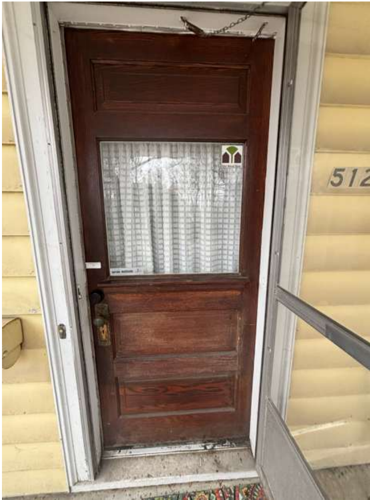
Existing Front Door
