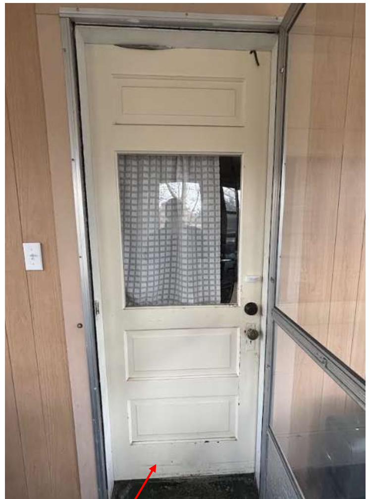
Existing Rear Door
