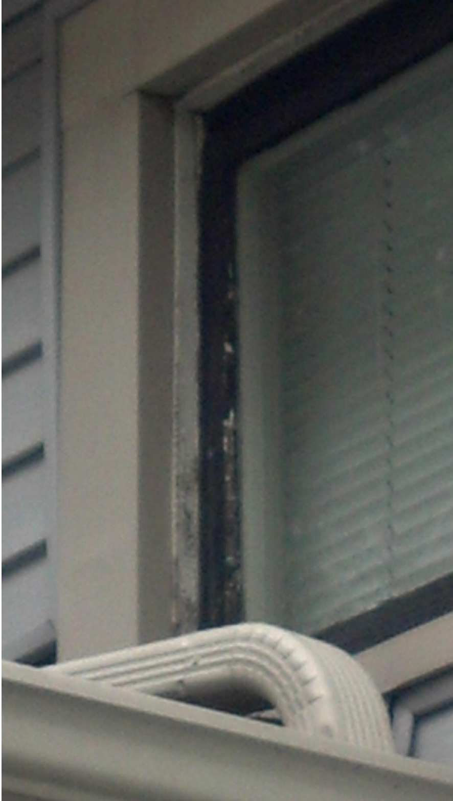
662 – Wood window with black storm, exterior
