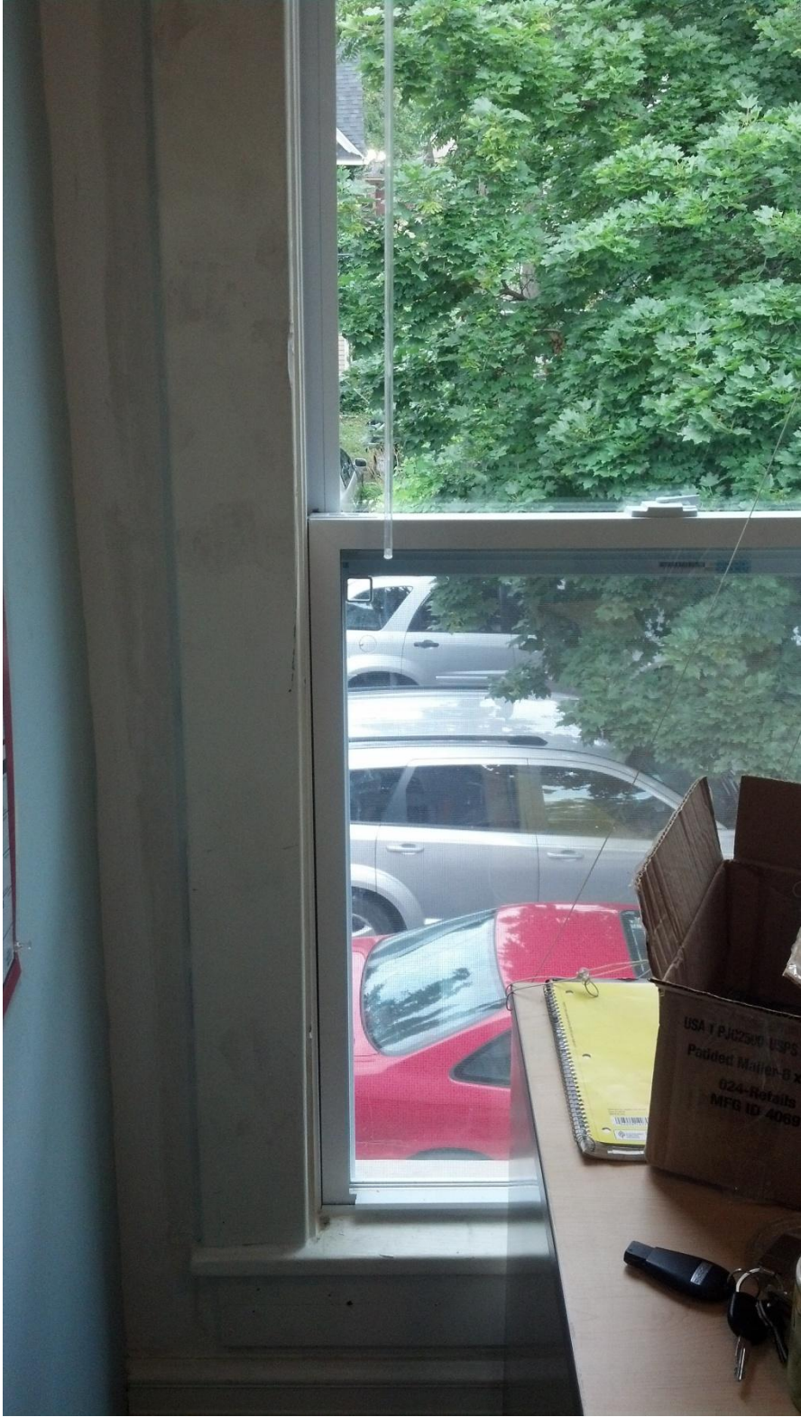
916 – New window upstairs, interior
