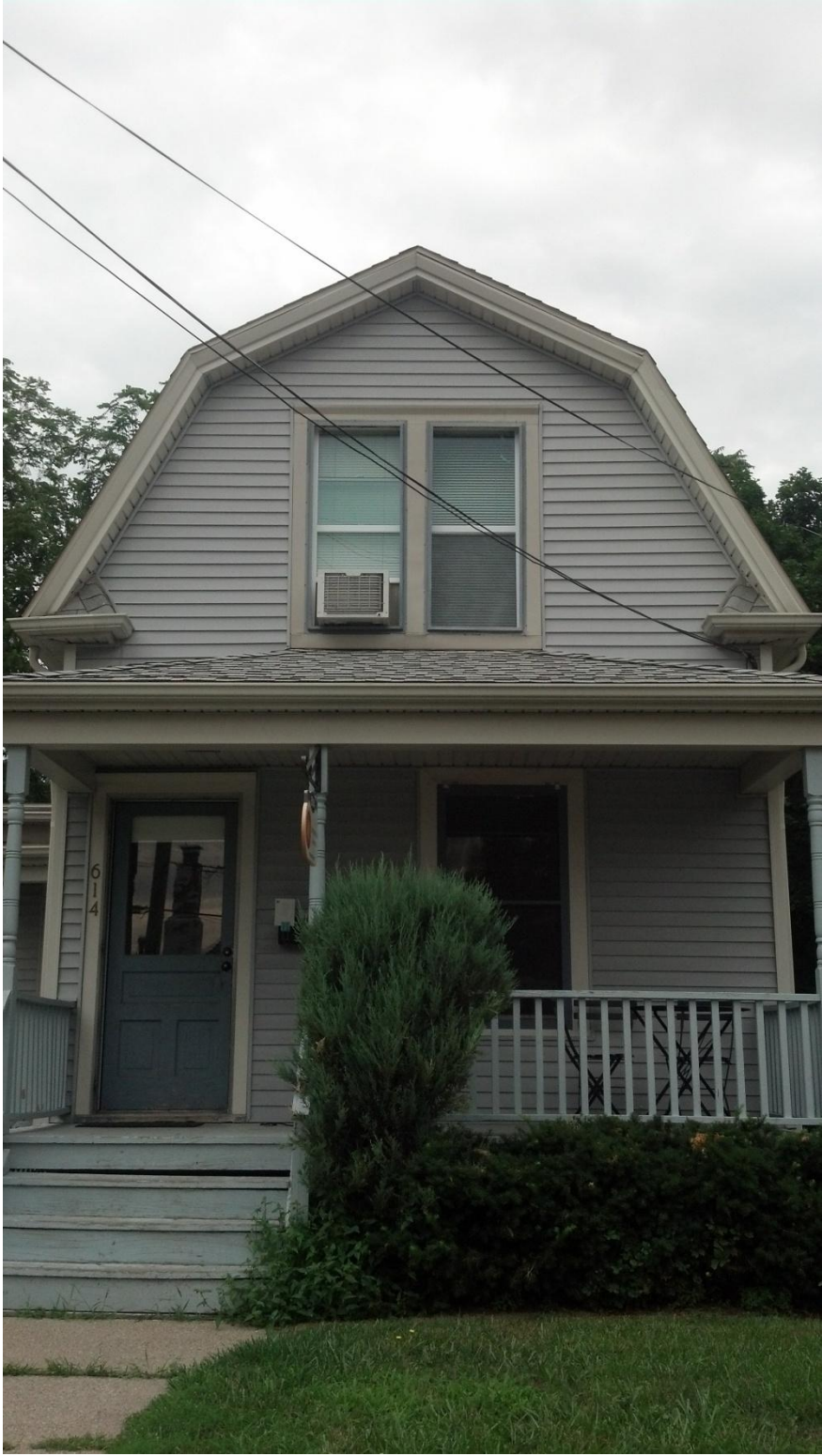
Photo 626 – front of house with new windows upstairs
