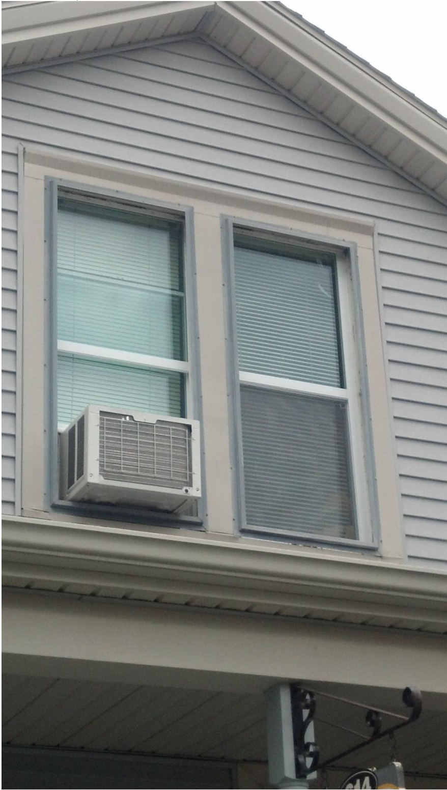
840 – New upstairs front windows, exterior
