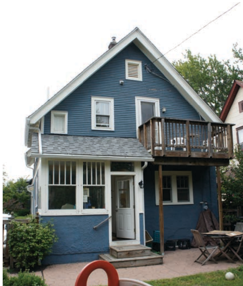
Photo of west elevation (deck to be removed) and new addition at right to be constructed
