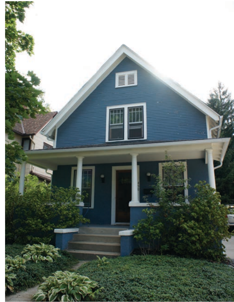
Photo of east elevation (no changes)
