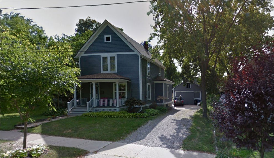
320 S Seventh Street (Aug 2017 courtesy Google Street View)
