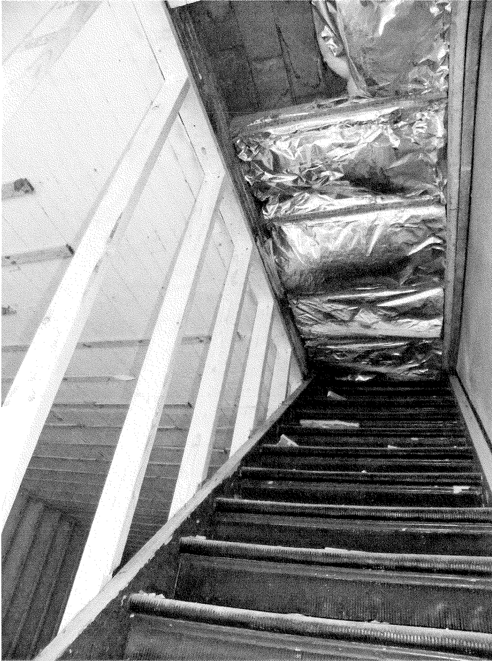
The original stairs to the former second and third floors still exist within the remaining single story Running Fit Building.
