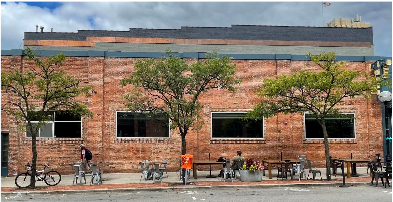
W LIBERTY ST. FACADE
