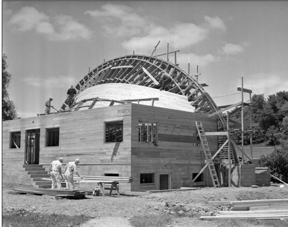
1938 Construction Dependent Wood Structures NOTE: Below grade door and windows
