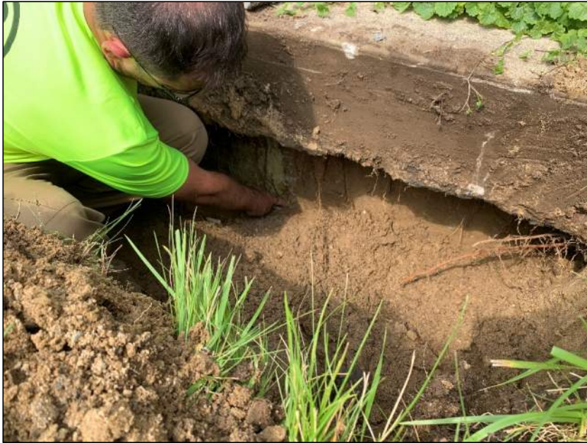
Photo 11: Along East Wall
