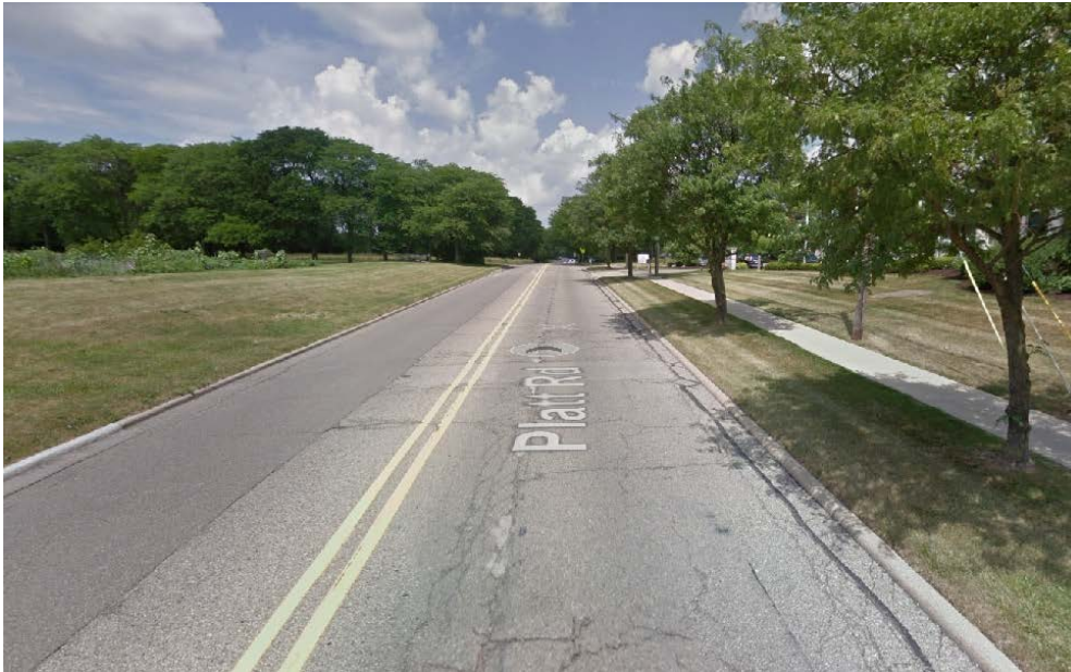
Existing Lane Configuration
