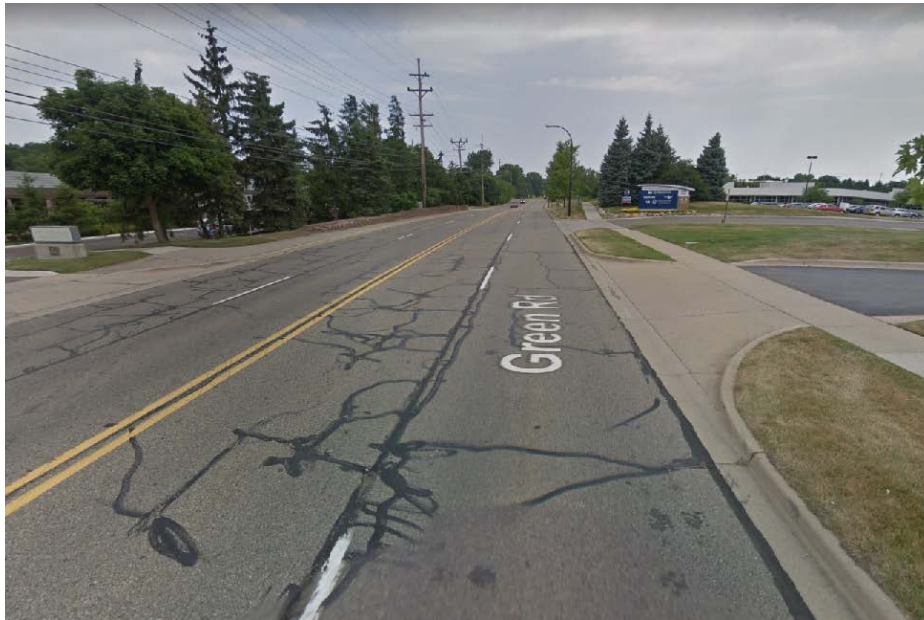
Existing Lane Configuration
