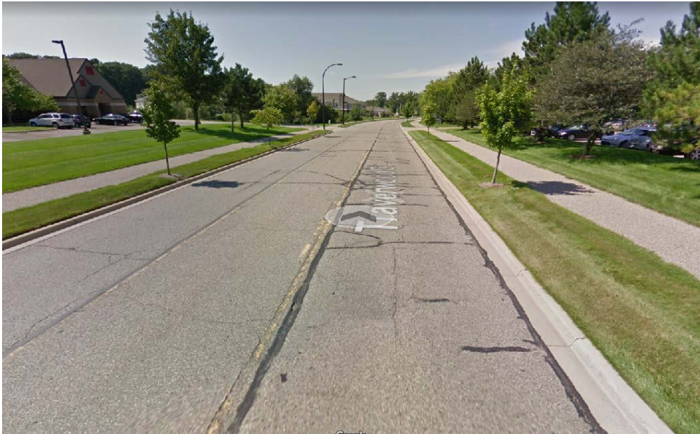
Existing Lane Configuration
