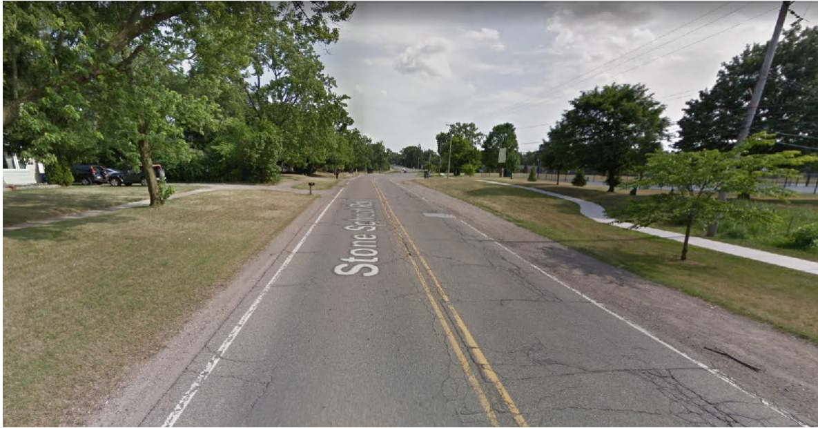
Existing Lane Configuration
