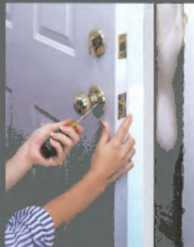
5. Install door hardware.
