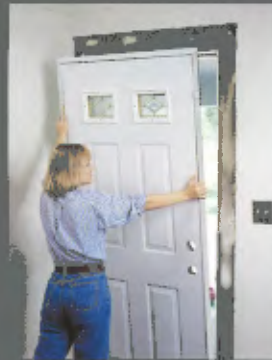
3. Insert new replacement unit into the opening from the interior of your home.
