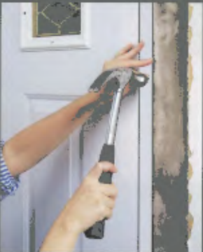
4. Nail replacement unit into position.
