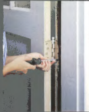
2. Remove the old door, strike plates, hinges and threshold.
