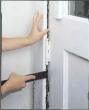
1. Carefully remove and save interior trim.
