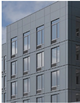
WINDOW WALL SYSTEM BLACK FRAMES WITH CLEAR LOW-E GLASS (SOLARBAN 60)
