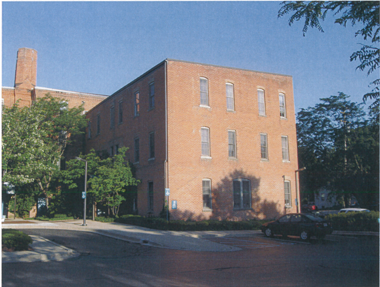
#1.6 August 12, 2011 Keck/Michigan Furniture Company North & east elevations (partial) View looking northwest
