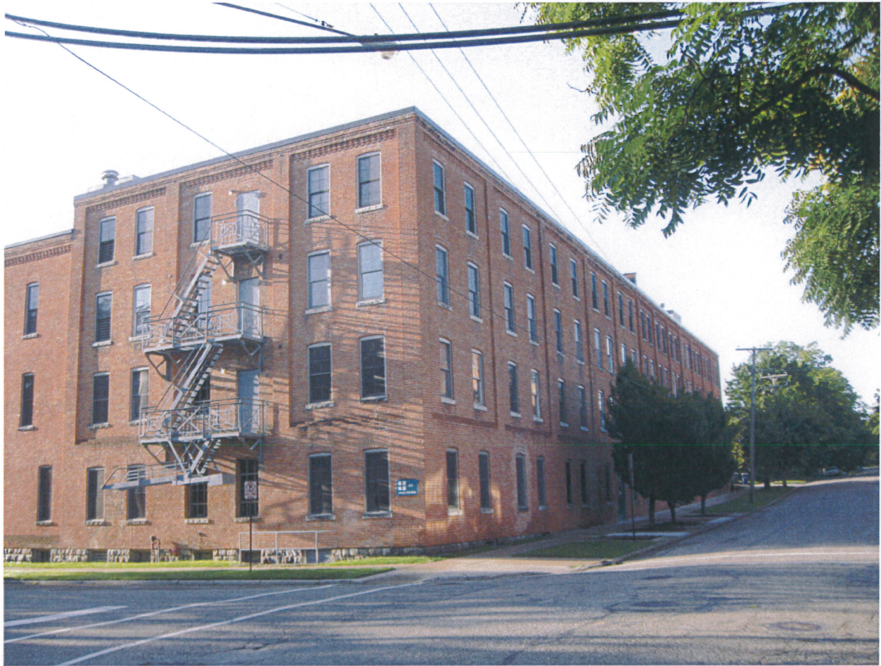
#1.8 August 12, 2011 Keck/Michigan Furniture Company North & west elevations (partial) View looking southeast
