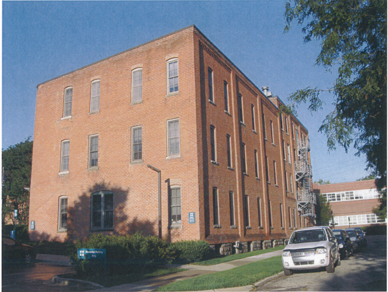
#1.7 August 12, 2011 Keck/Michigan Furniture Company East & north elevations (partial) View looking southwest
