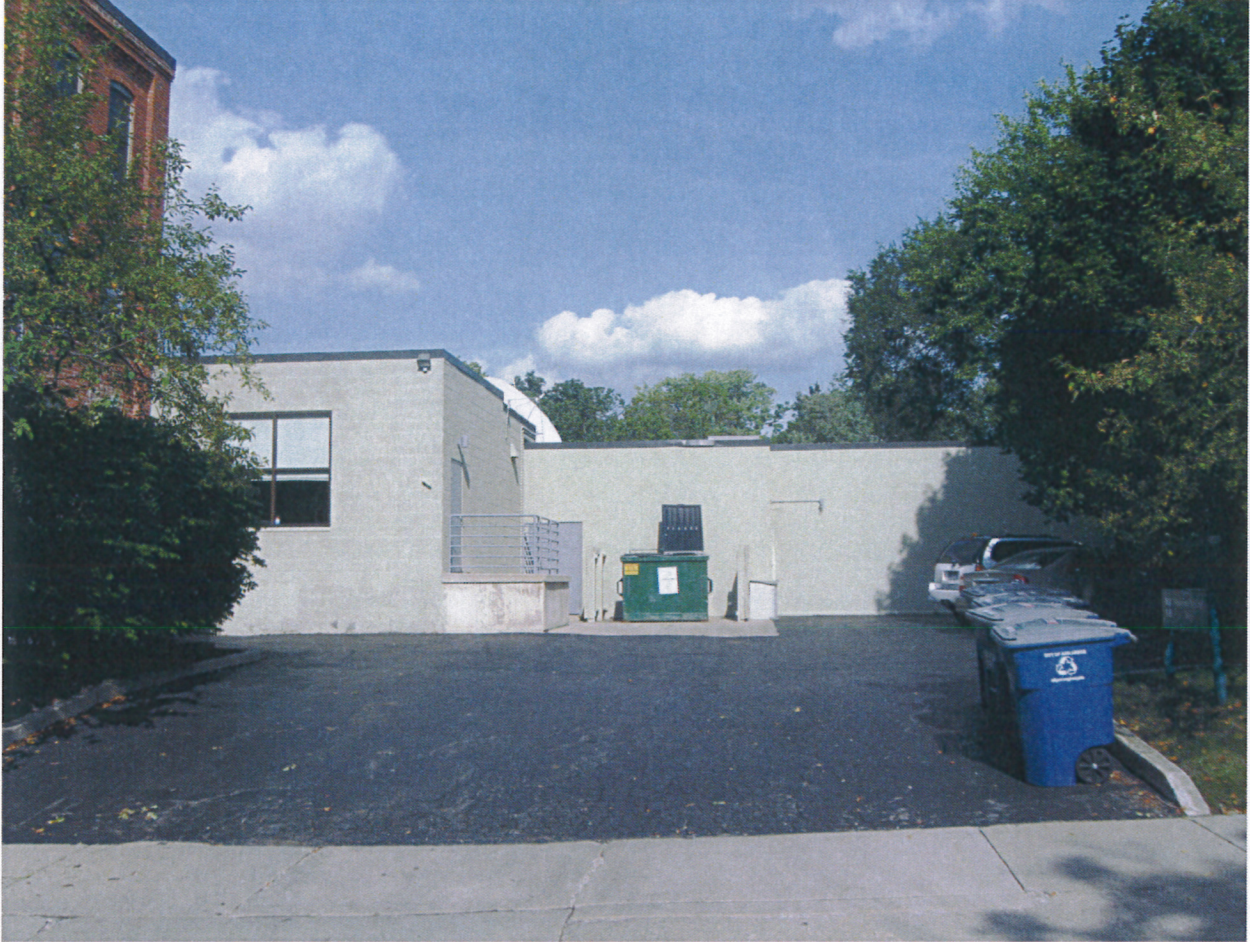
#1.12 August 12, 2011 Keck/Michigan Furniture Company West elevation (partial) View looking east
