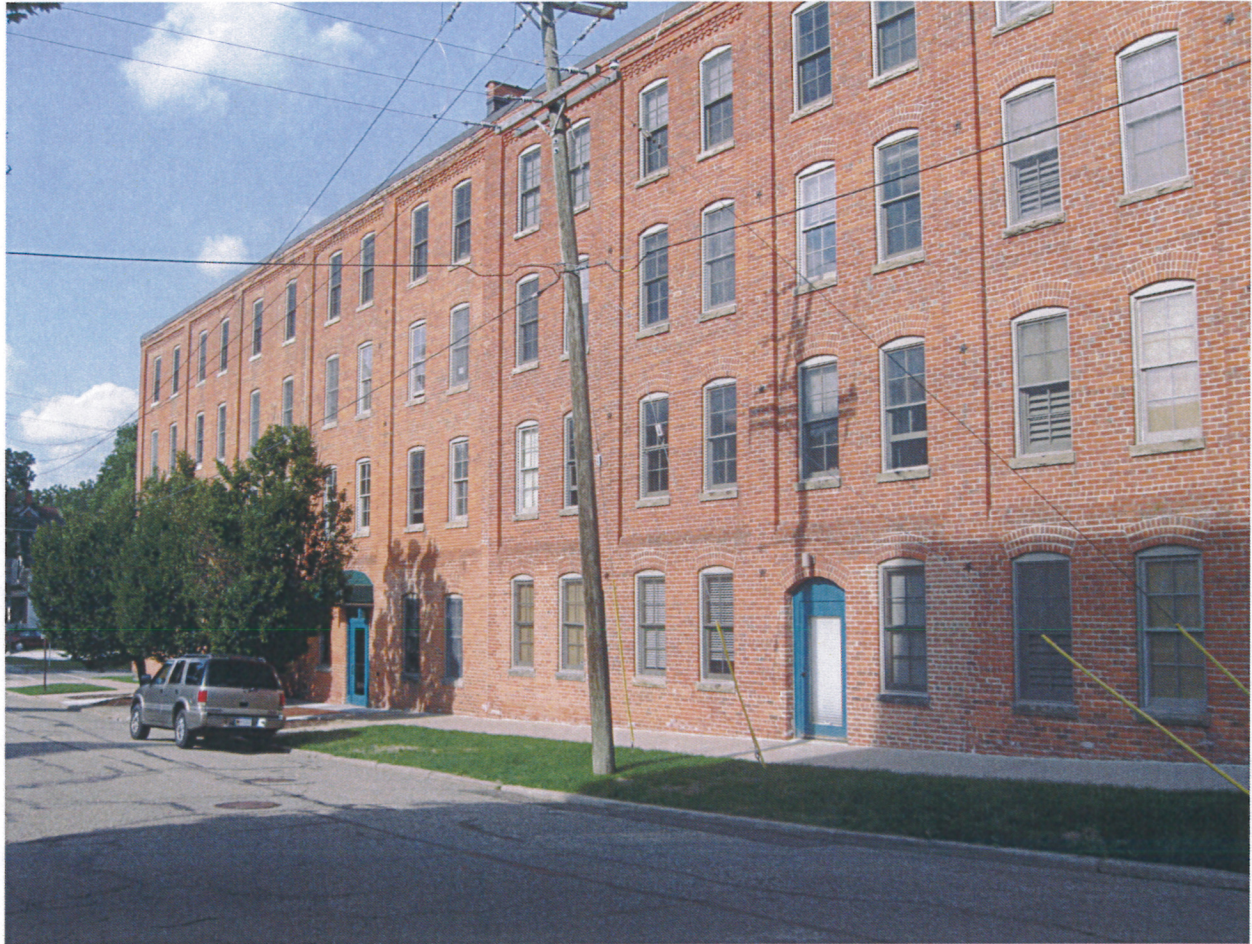
#1.9 August 12, 2011 Keck/Michigan Furniture Company West elevation (partial) View looking northeast
