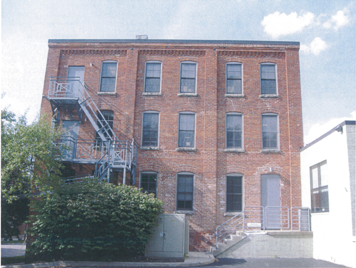
#1.11 August 12, 2011 Keck/Michigan Furniture Company South elevation (partial) View looking north
