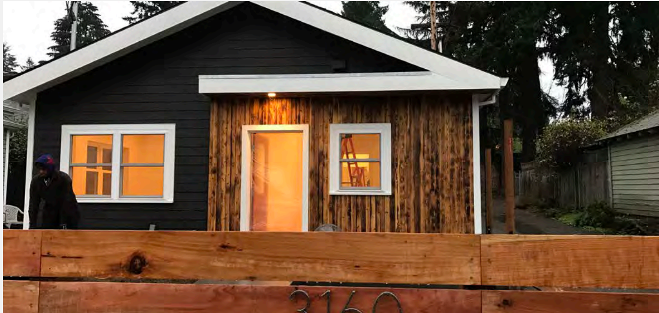
New Construction ADU for mom in the kid's backyard!
