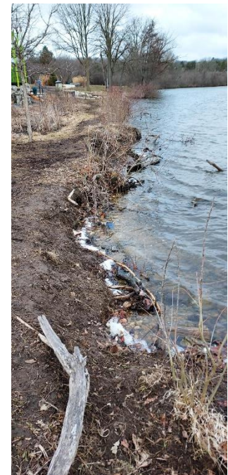
Photo 4: Shoreline about 30 feet from buffer facing West
