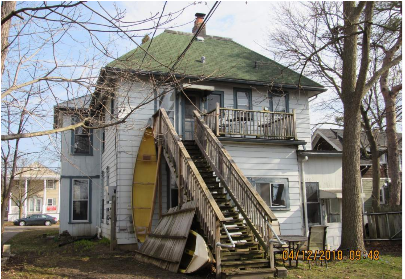
Rear of House
